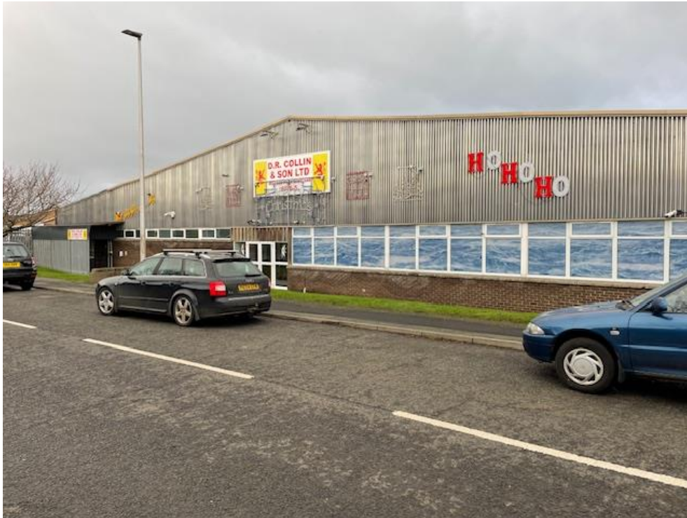
Image showing the South Facing elevation of Shed 5 factory onto Eyemouth Industrial Estate.
