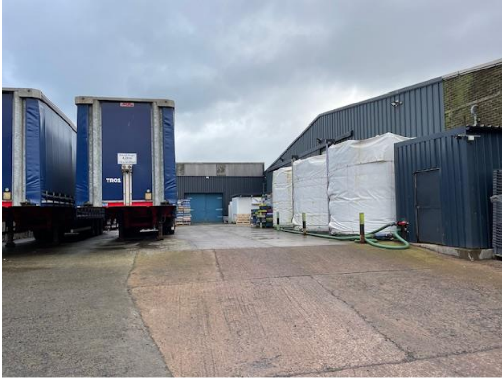
Image showing the North facing elevation of the factory.
