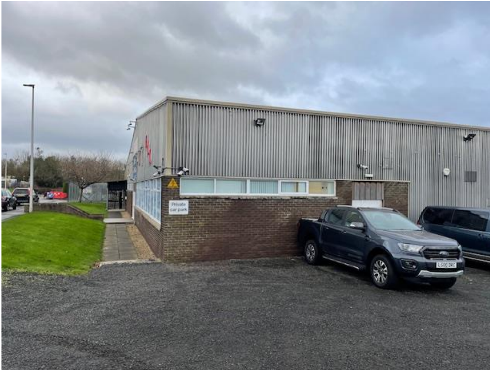
Image showing the South-East corner of the factory
