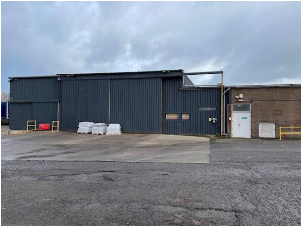
Image showing West facing elevation of the factory.
