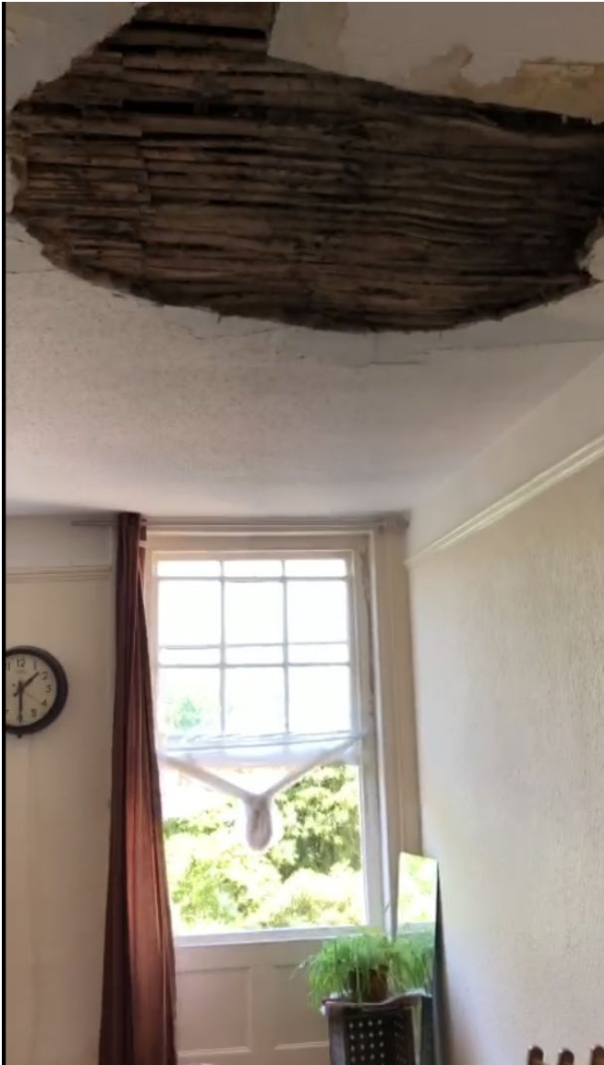
View towards existing sash windows & ceiling
