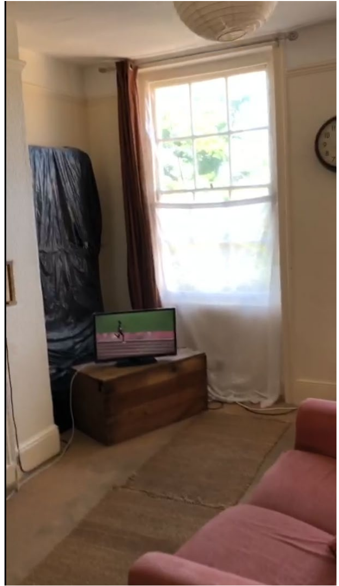
View towards existing sash windows & chimney
