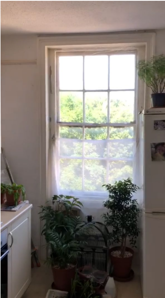
View towards existing timber sash window within Kitchen
