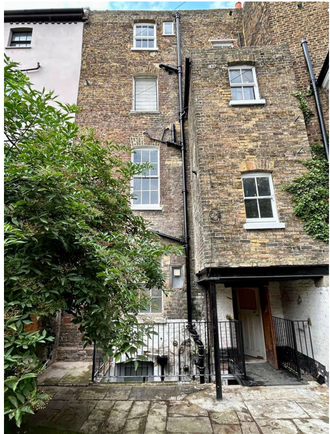
Existing view of rear elevation
