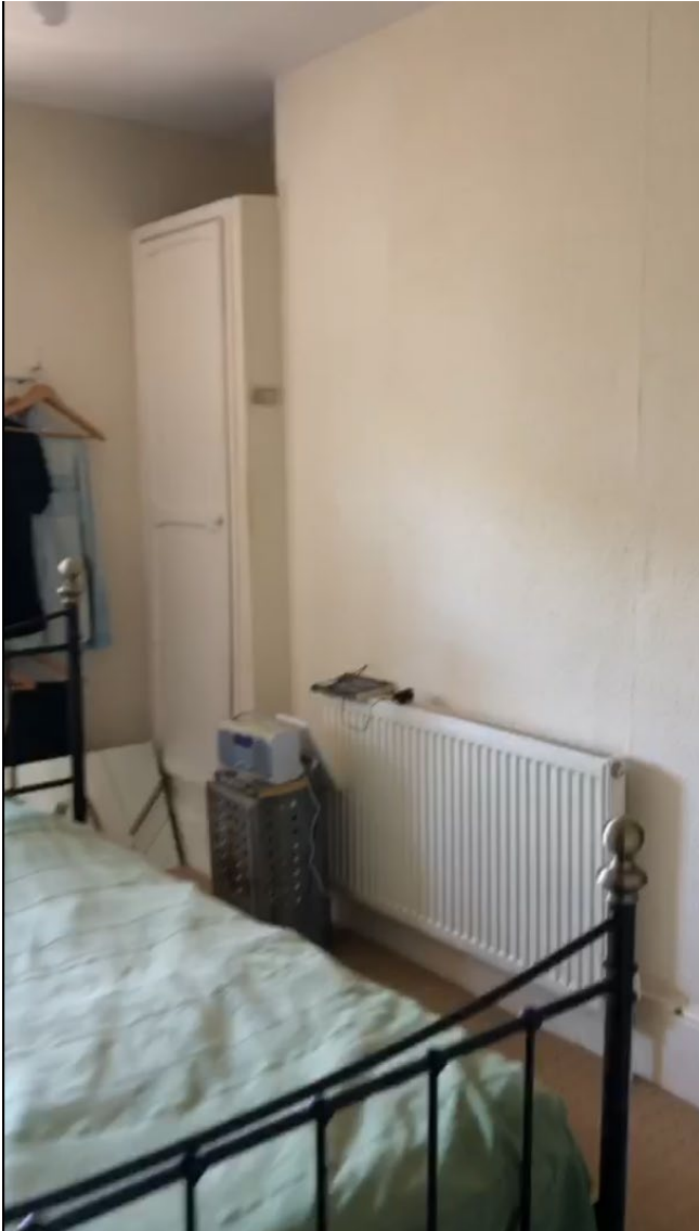
View towards existing chimney breast within bedroom
