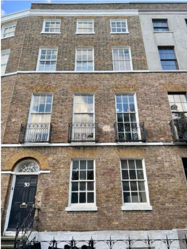
Existing view of front elevation
