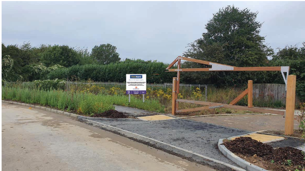
Figure 7: View of the car park showing signage D
