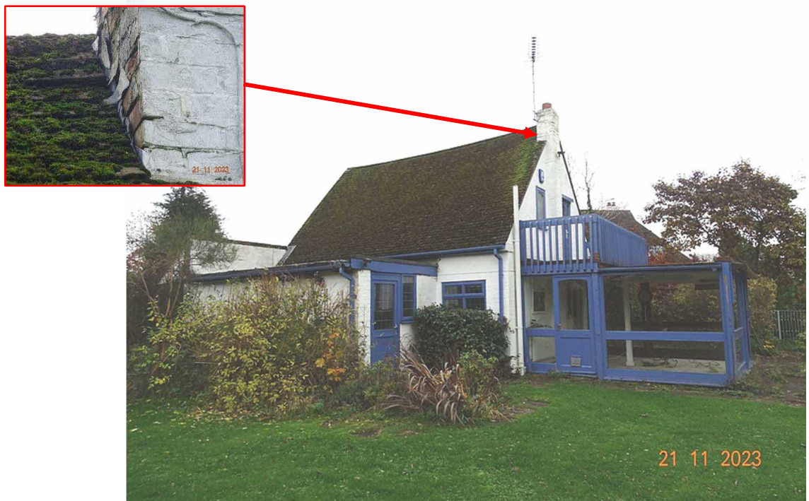
Plate 2 | Describing north side of cottage from CP(B) Inset phot showing loose flashing.
