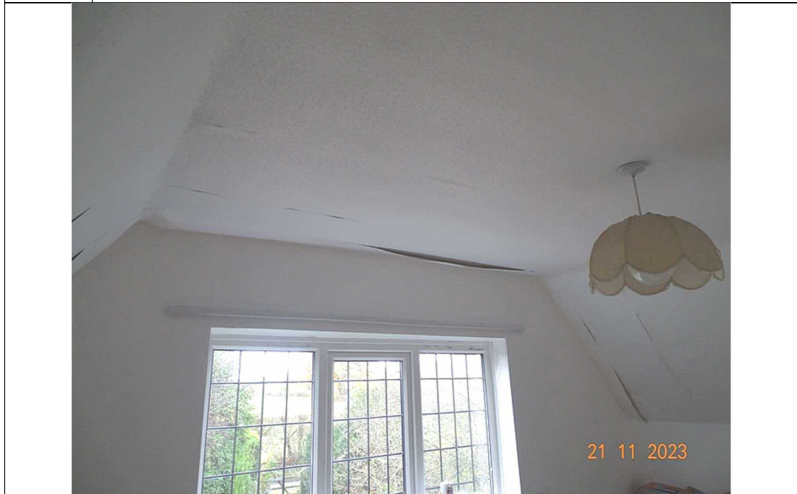
Plate 6 | Describing internal vaulted ceiling inside 1 st floor of cottage.
