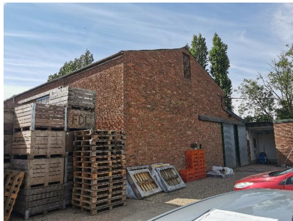
External view of the brick building
