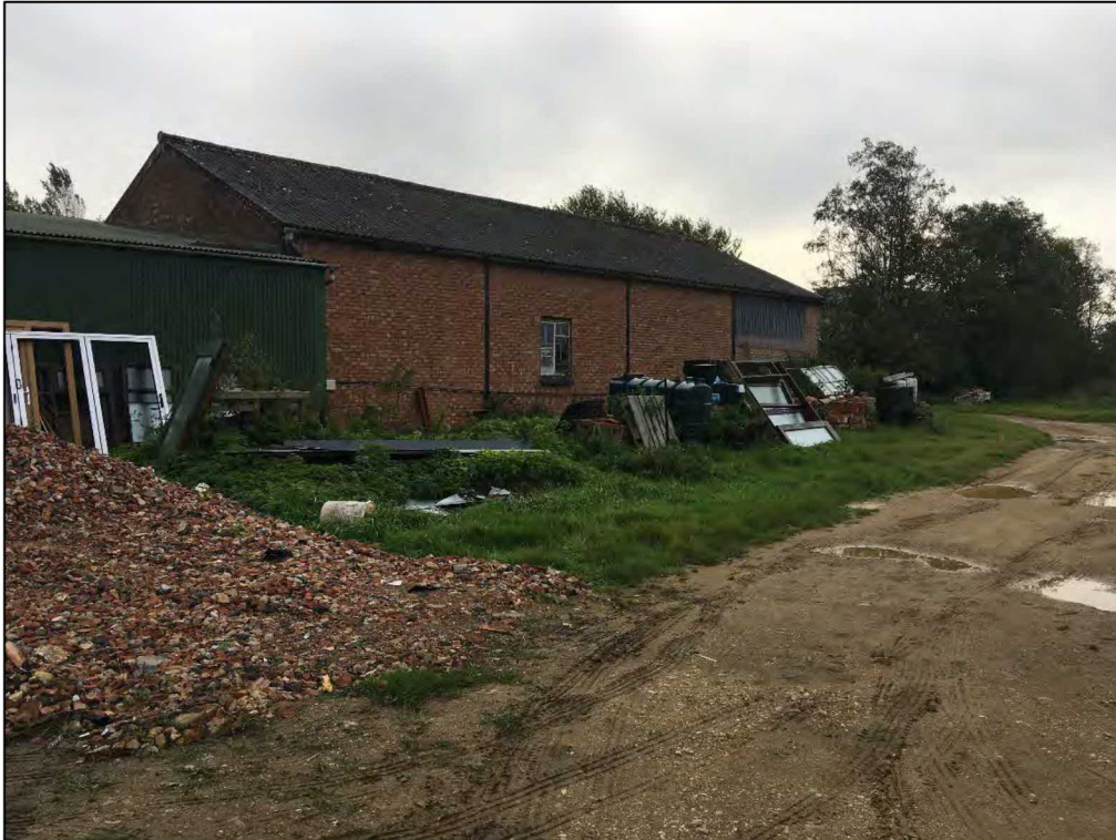
Photograph 7: The rear / western elevation of the building on-site and track.
