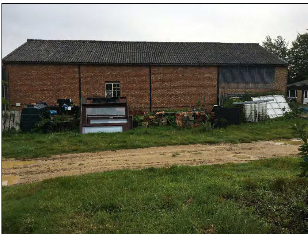
Photograph 6: The rear / western elevation of the building on-site.
