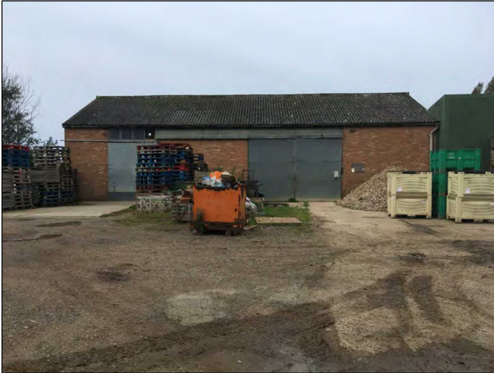
Photograph 1: The building on-site – its eastern side.
