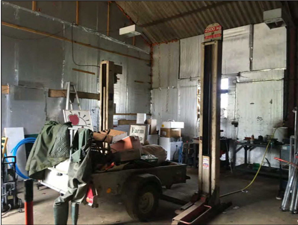
Photograph 3: Inside the storage unit. The insulating board acted as a partition wall between the two units.
