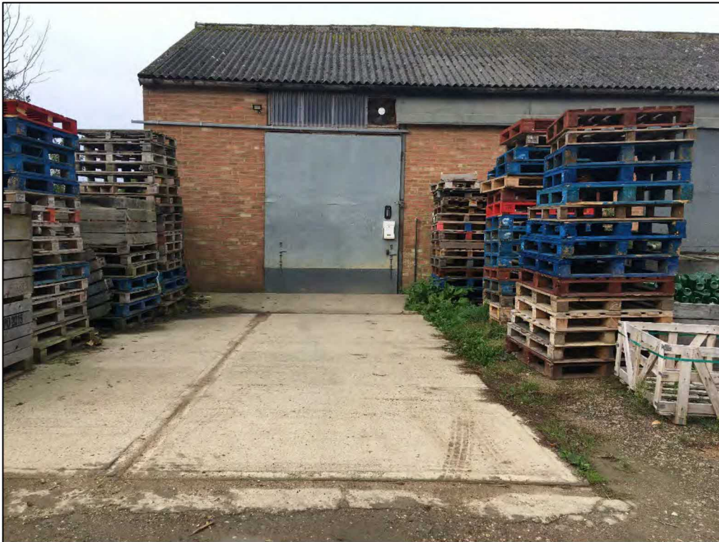
Photograph 4: Entrance to the left hand / southern unit, which was in use for the storage of fruit and vegetables.
