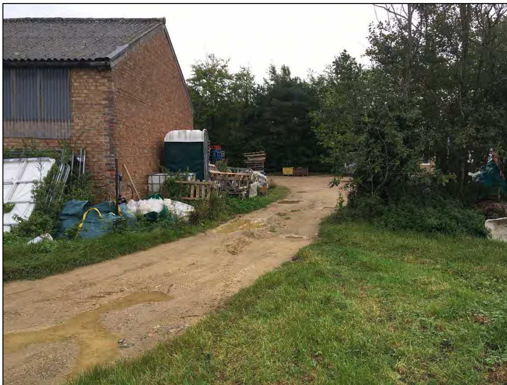
Photograph 5: The southern end of the unit, together with an access track.
