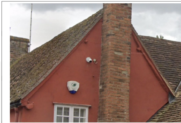
1 - View showing the current state of the roof
