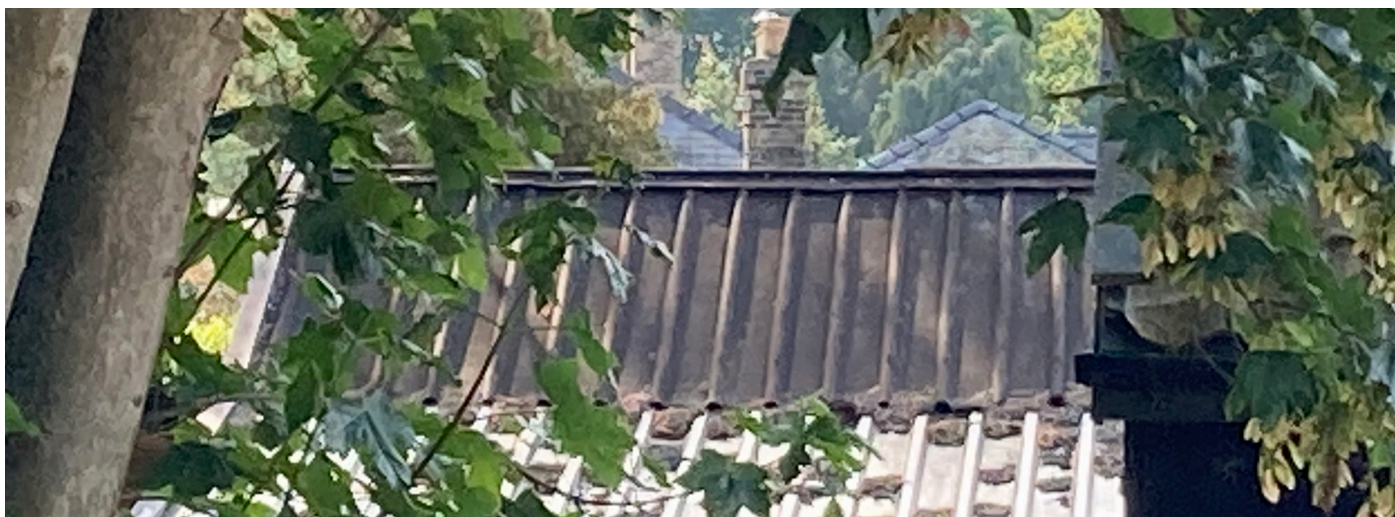
Fig.7 Existing zinc roofing on adjacent outbuildings
