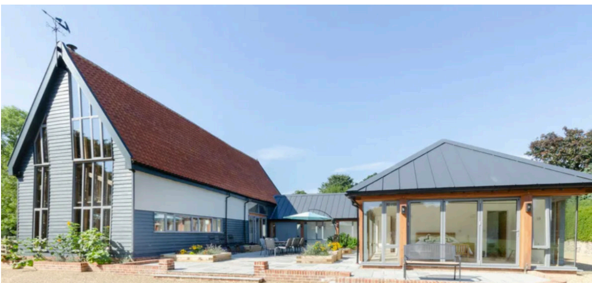
Fig.2 Example of metal windows and bi-fold doors in a nearby barn conversion
