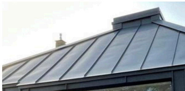
Fig.6 Example of a similar zinc roof
