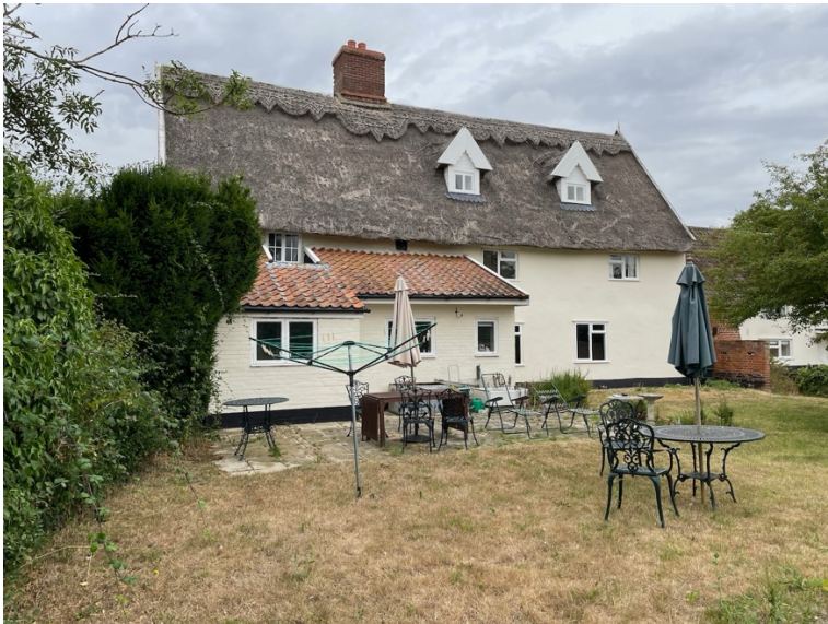
South elevation showing use of clay pantiles on the existing extension
