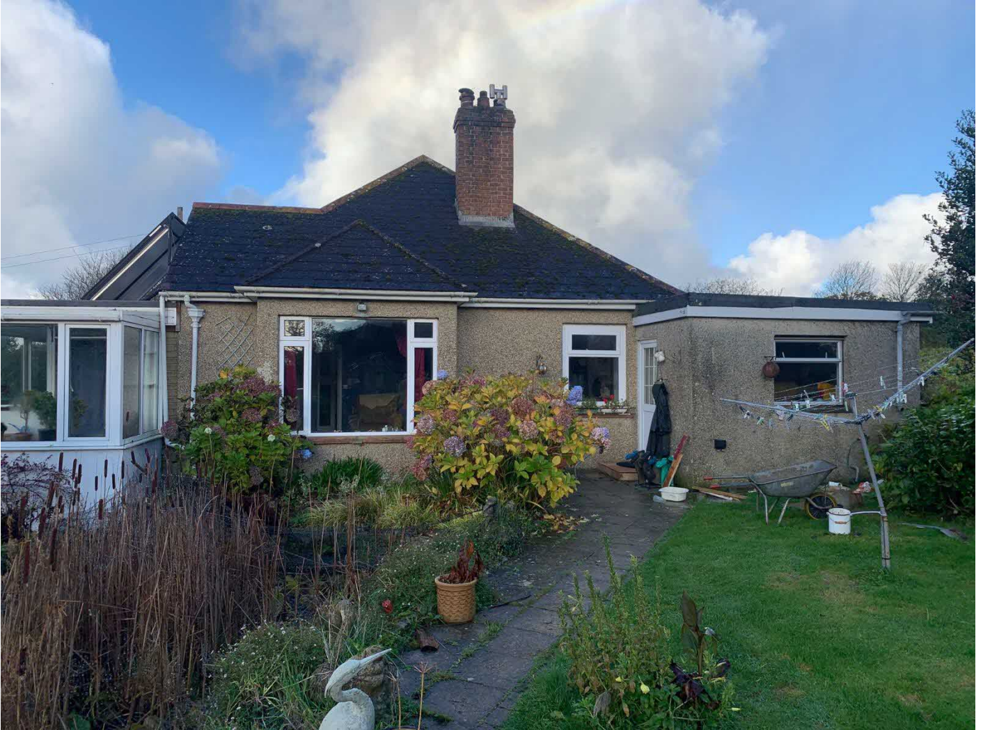
Figure 1: South-eastern elevation of building
