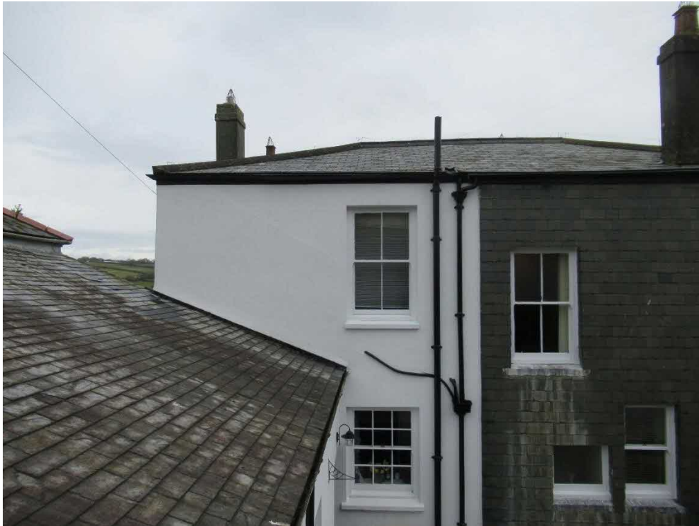
South West elevation showing approved position of solar panels and low pitch of existing roof.
