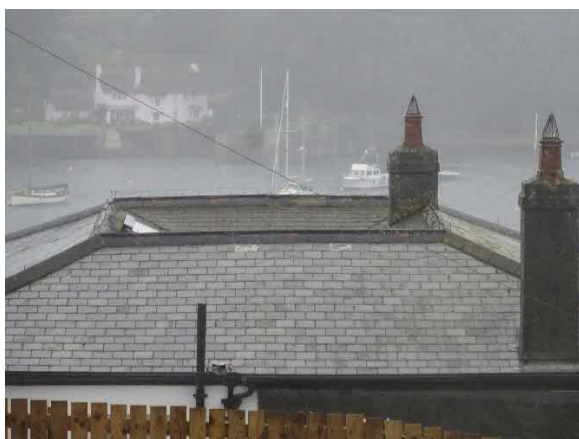
Inner roof valley as seen from within site boundary.
