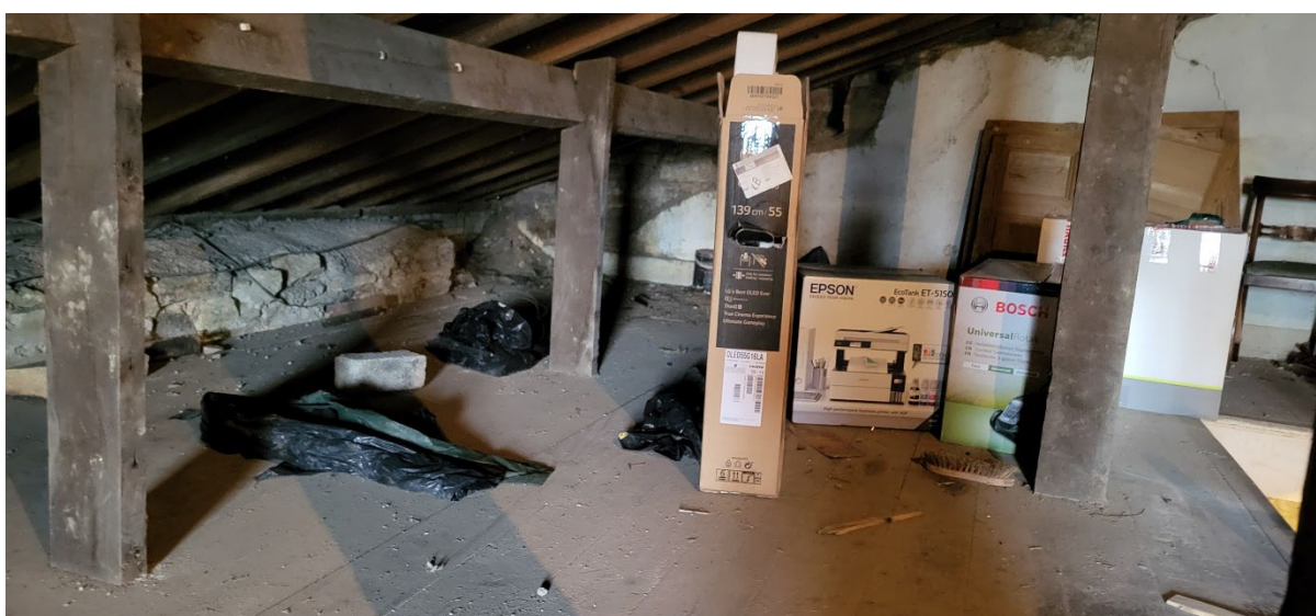
Figure 12: Interior of the roof space of the annexe
