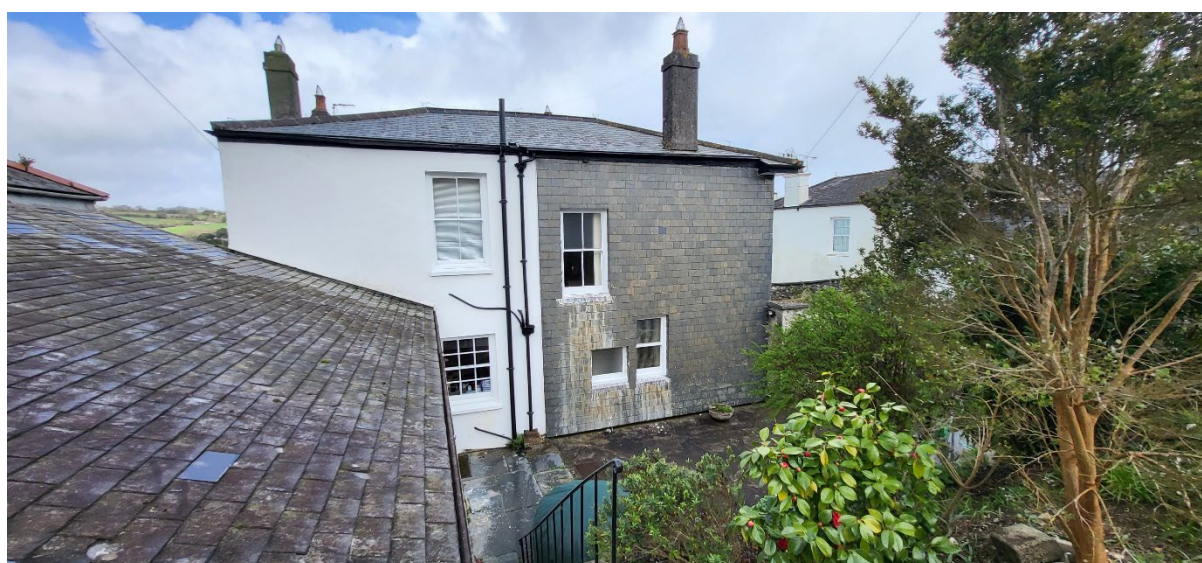
Figure 2: West elevation of 12 Stratton Terrace
