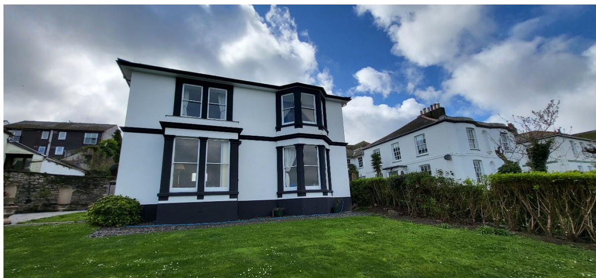
Figure 1: 12 Stratton Terrace; Grade II listed Georgian Villa, east elevation
