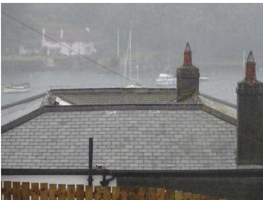
Inner roof valley as seen from within site boundary.
