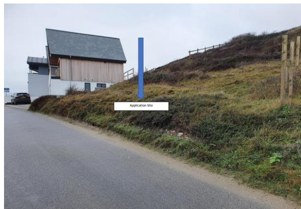
Fig.4 – Application site looking west.
