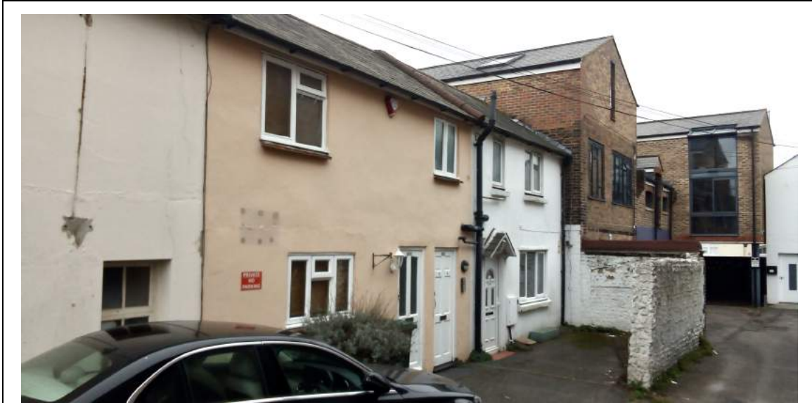
The row of adjoining mews houses, Nos. 221B and 223B to the south, with taller commercial mews buildings beyond. Remnant of flint wall around 221B
