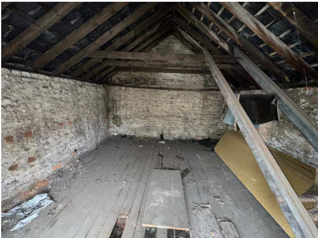
The First Floor, looking south.
