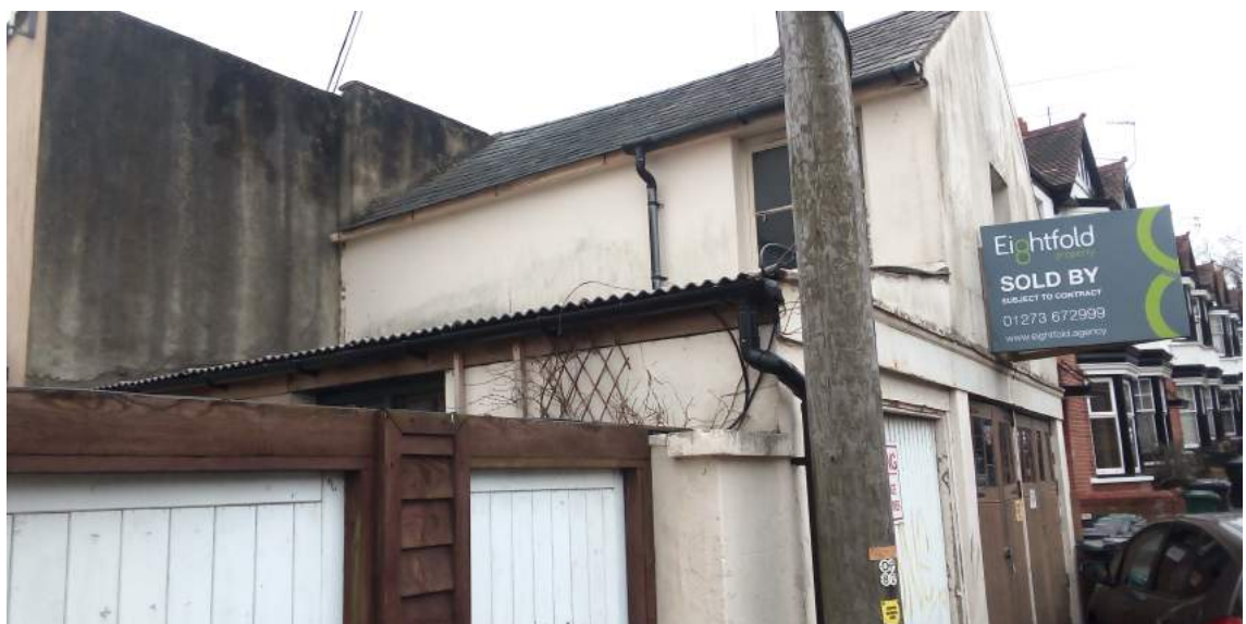
The East Elevation, facing the rear of 225 Preston Road.
