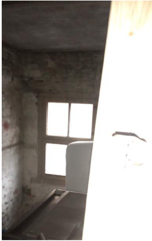
The west wall, southern window.
