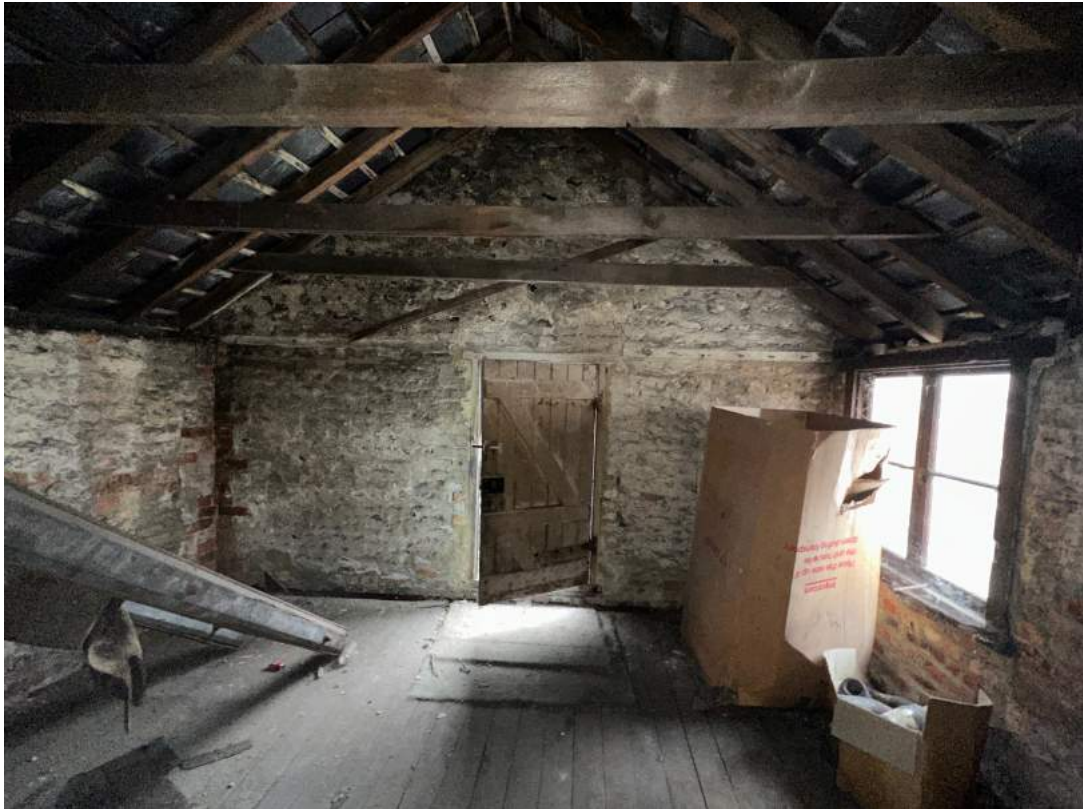
The First Floor, looking north.
