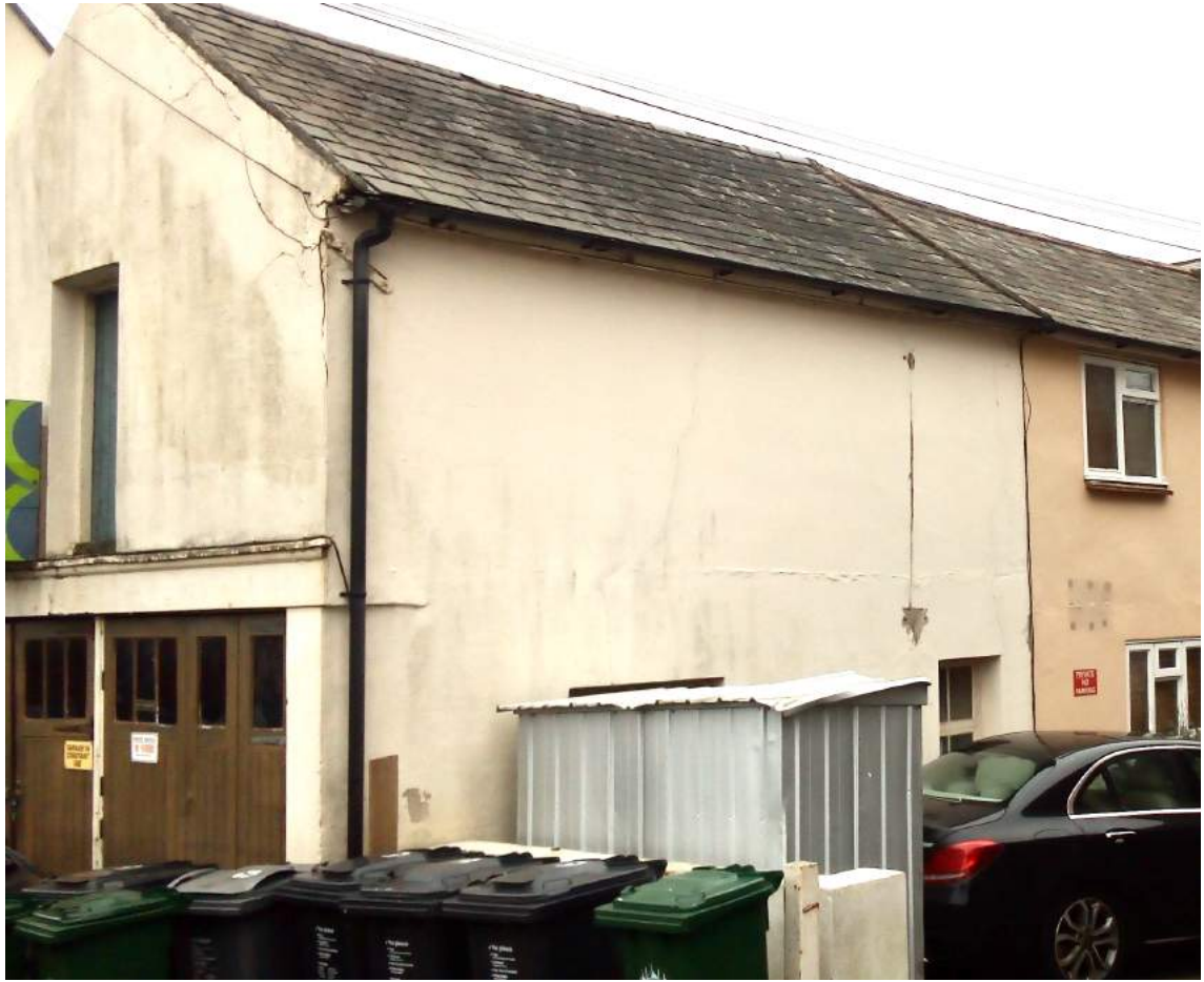
The west elevation onto the mews.
