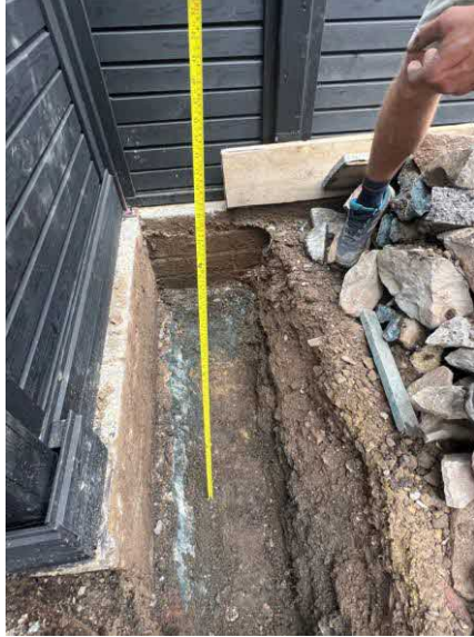
Image 1 – Trench dug to >600mm for tree planting.
