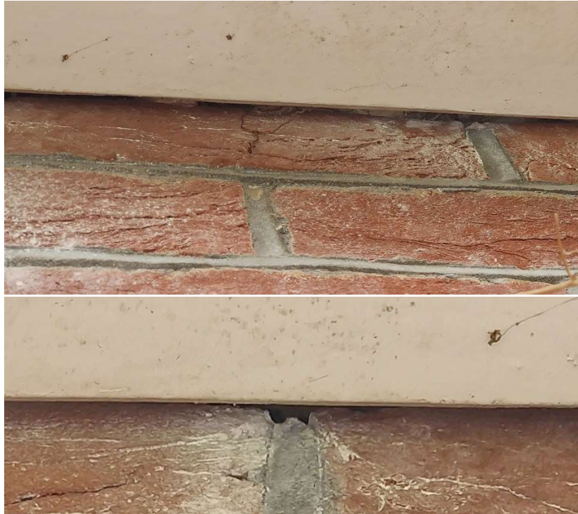
Figure 9. Internal gap under the eaves (November 2023).
