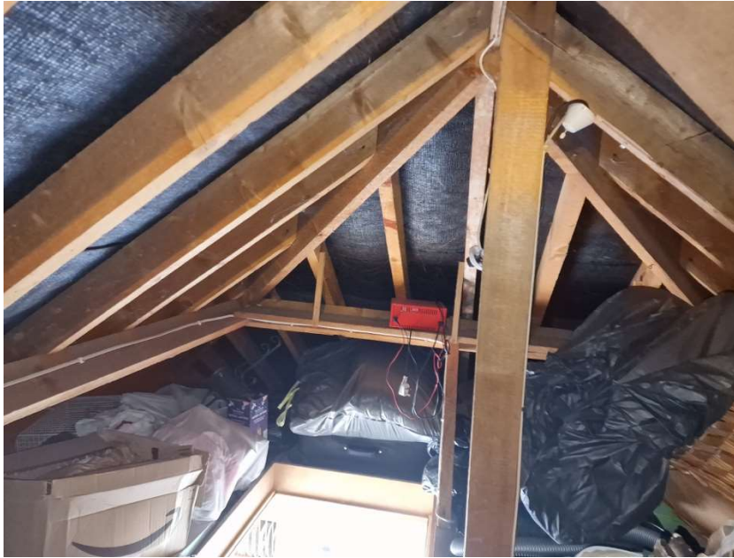
Figure 6. Internal view of the loft space within West Wadlington’s kitchen (November 2023).
