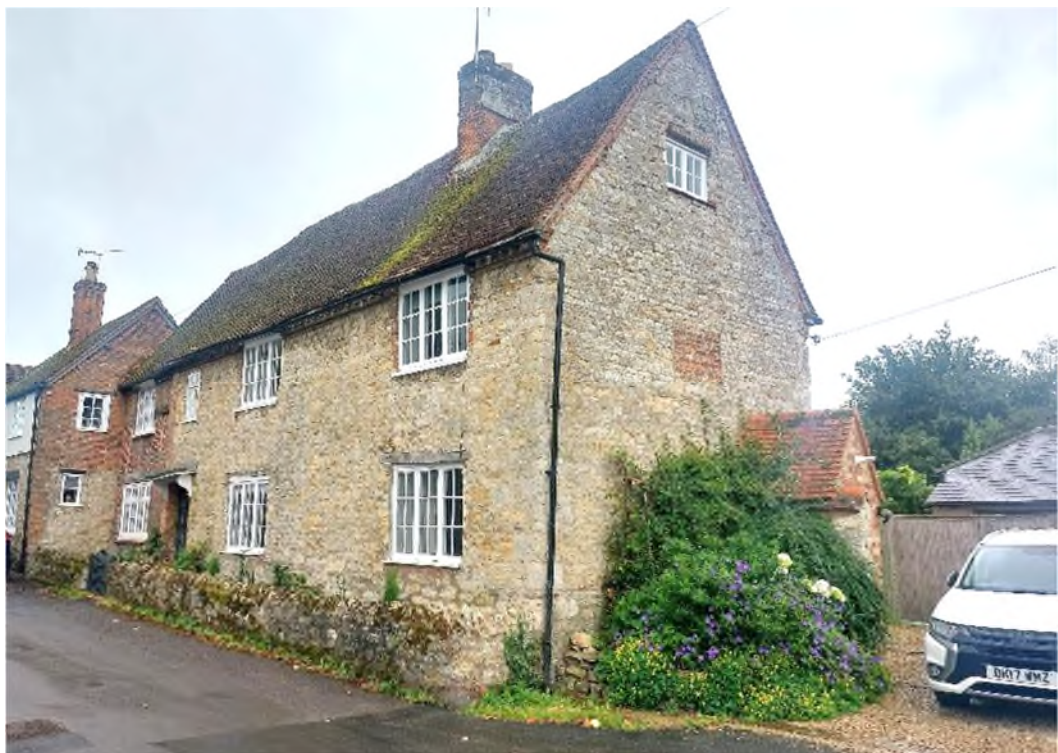
Figure 1 Front and north gable elevations of The Old Post.
