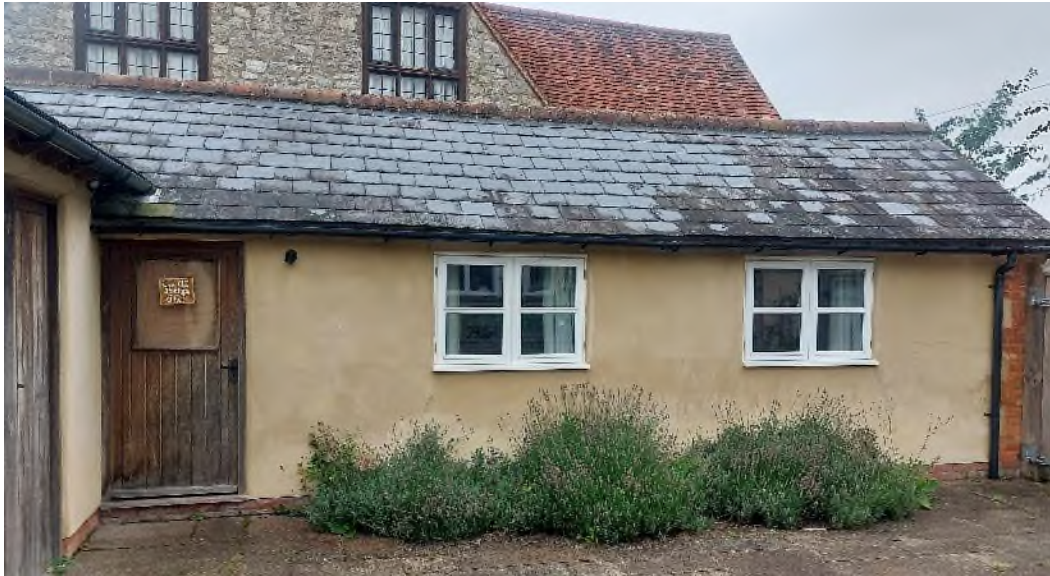
Figure 3 The front elevation of the outbuilding.
