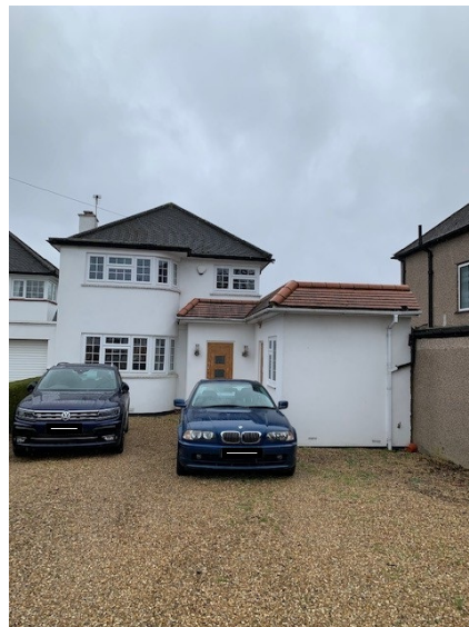
Existing Street Frontage 57 Hale Drive
