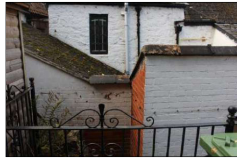
PHOTOGRAPH OF WALLS WHERE VENTS PROPOSED
