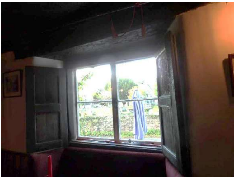
Original frame/inserted C20 casements [Window nearest the fireplace]
