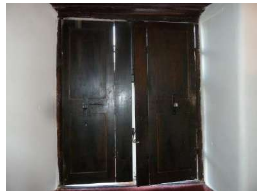
Later circa C19 early C20 machine cut timber shutters
