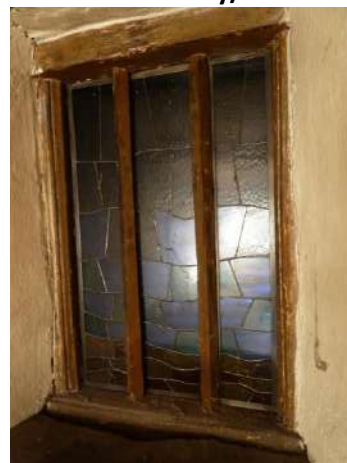
Recessed blocked window x3 slim square mullions set diamond-wise in the frame suggesting the type of early C17
