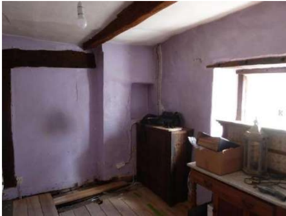
Recess in side wall above cupboard below in bar
