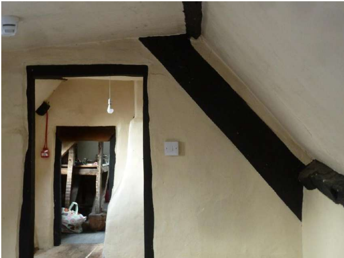
Lime plaster to walls/lath & plaster ceiling, exposed purlin
