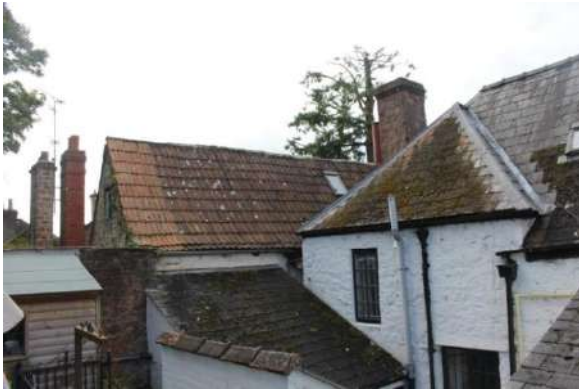
View towards Dower Cottage and Pantiled roof
