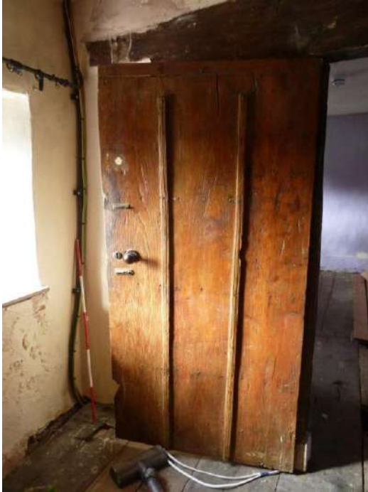
C17 Plank door To Front Bedroom
