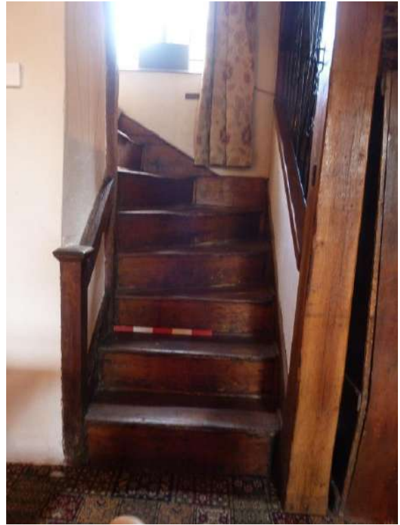
Late C17 Early C18 Timber Stairs to FF [50cm scale pole]
