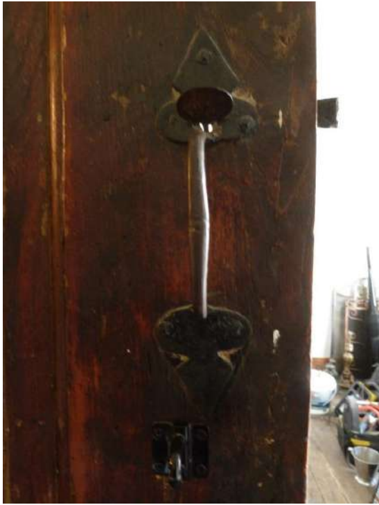
C17 doors with ironmongery
