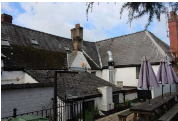
View towards wing of Lynchgate Cottage
