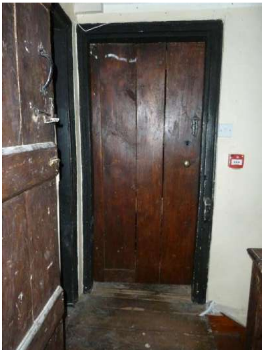
The 3 rd plank and batten C17 door
