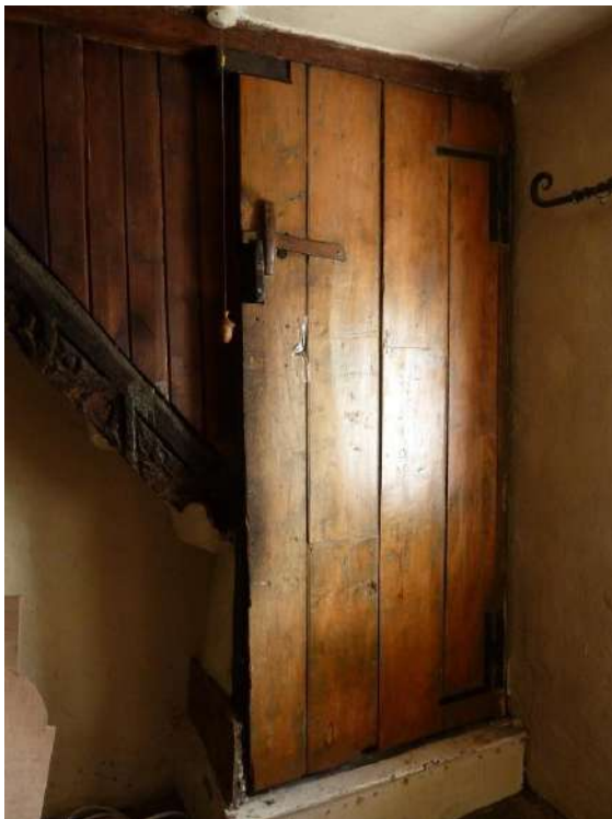
Plank and batten door to stairs
