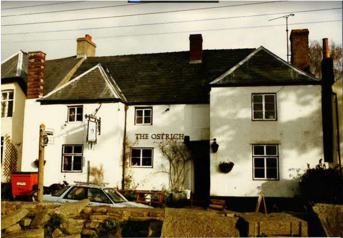
1992 front From HER ref 232 8 /63 date 25 /11/ 92 Buildings At Risk Register
