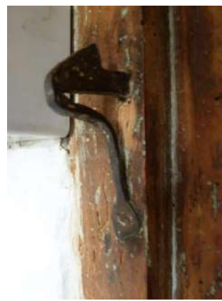
C17 doors with ironmongery
