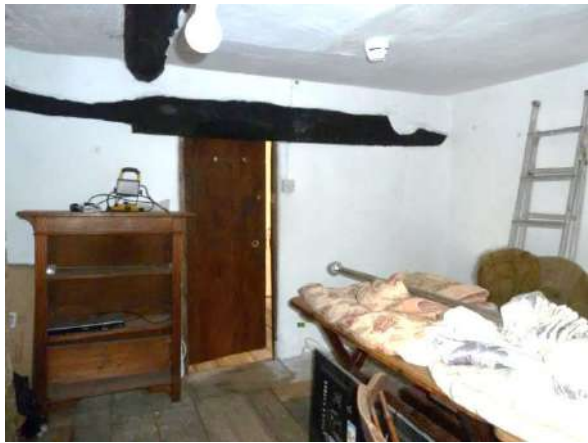
Exposed Beams and Timbers/Lintel to door.
