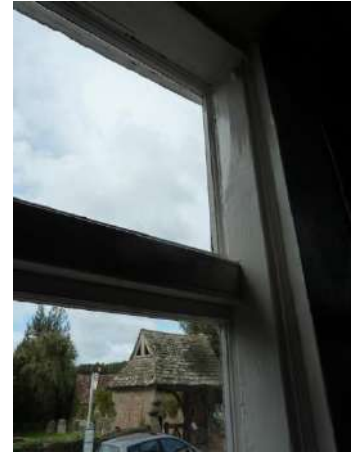
Original Window Frame and transom C17 or Early C18
