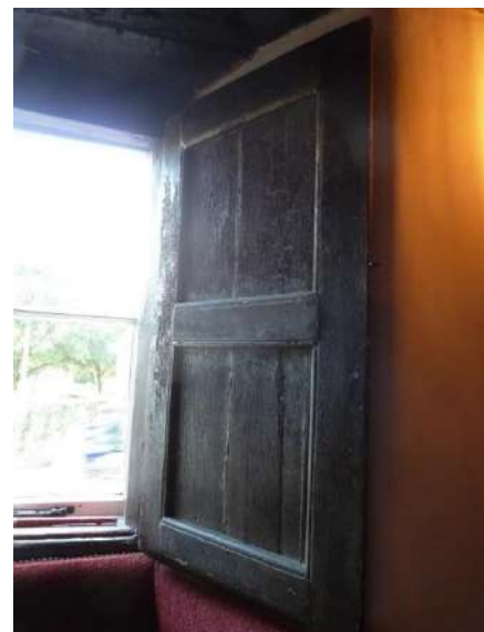
Original C17 Shutters [Window nearest the fireplace]
