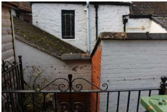
Rear of Toilet blocks
