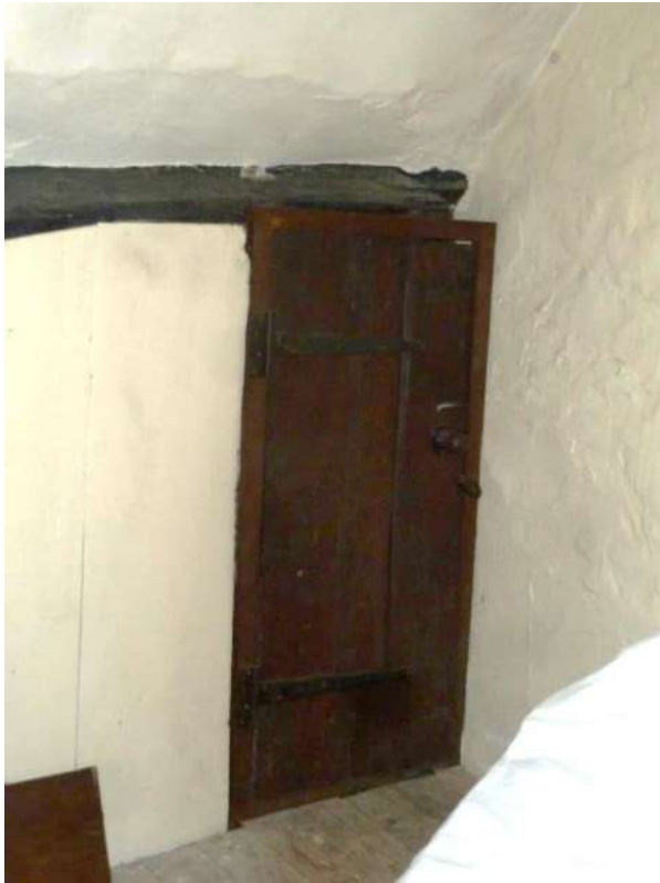
Half size C17 Plank door with applied vertical fillet mouldings [Later hinges]
