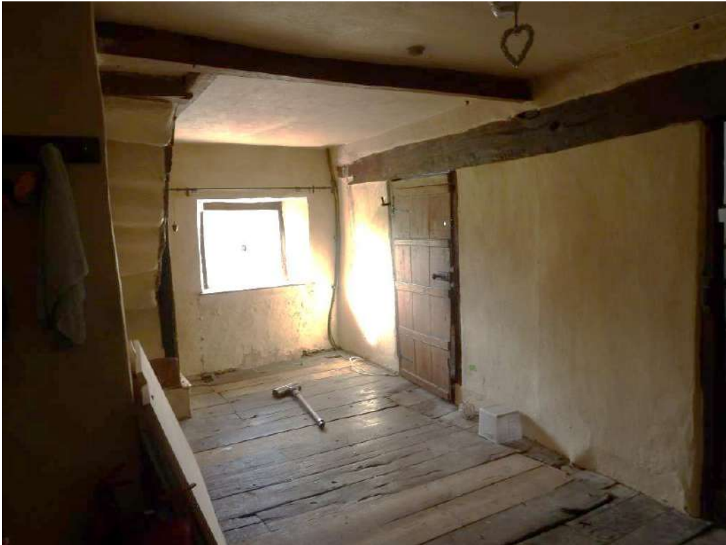
A large landing is above the main Bar below
