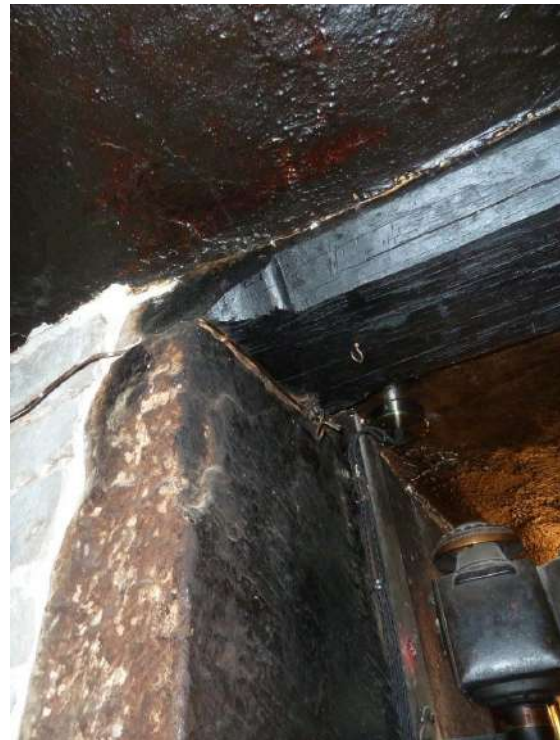
Chamfered Beam and stop resting on large C17 fireplace stone lintel
