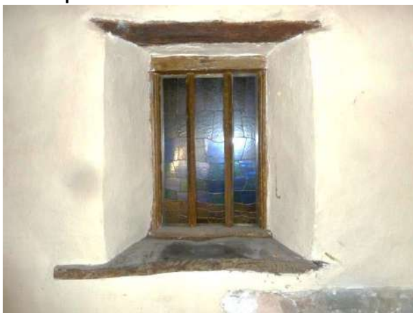
Recessed blocked window x3 slim square mullions set diamond-wise in the frame suggesting the type of early C17
