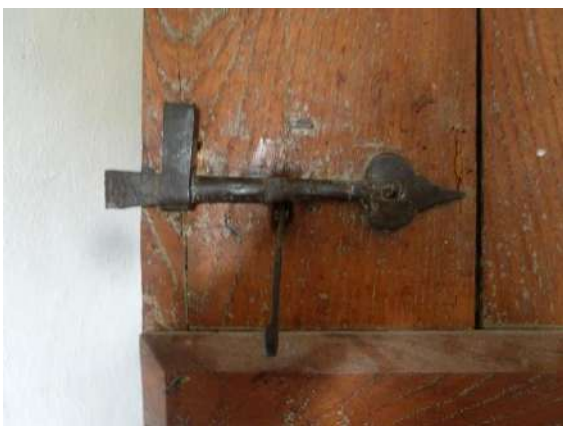
C17 doors with ironmongery
