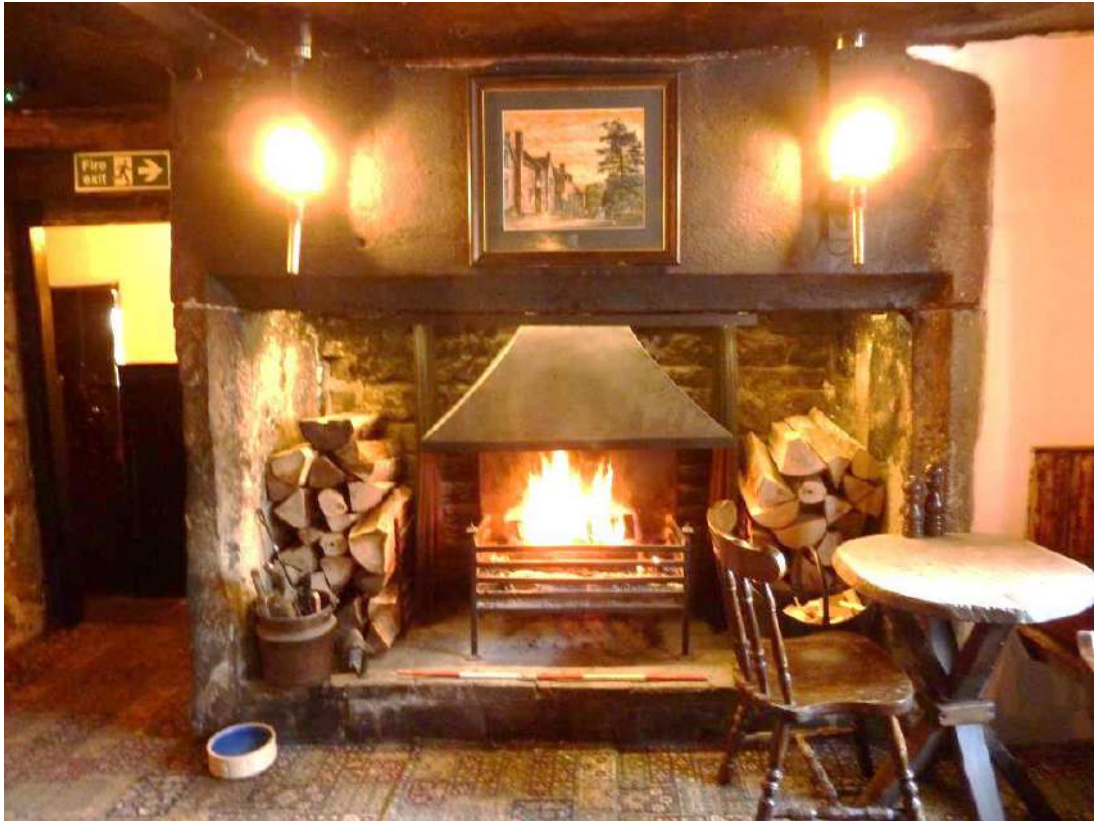
C17 Fireplace with large stone lintel with chamfer
