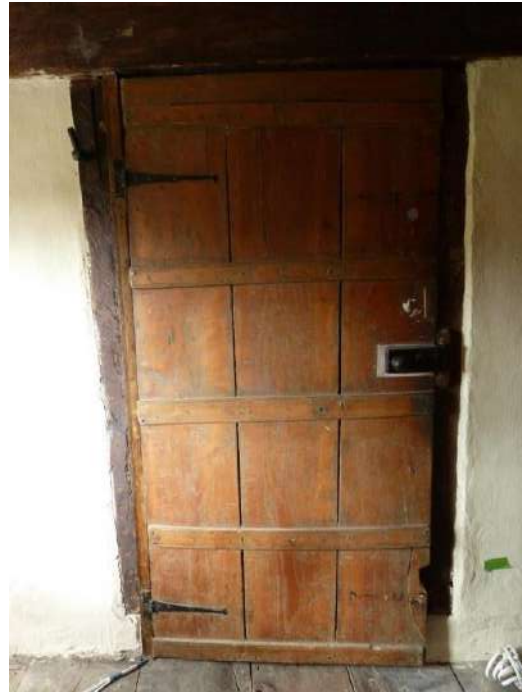
C17 Plank Rear of door to Front Bedroom
