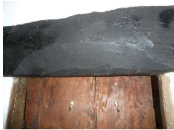
Exposed Beams and Timbers/Chamfered Lintel to door.
