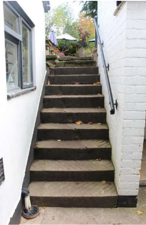
Concrete steps 1979 or 1939? To Gardens
