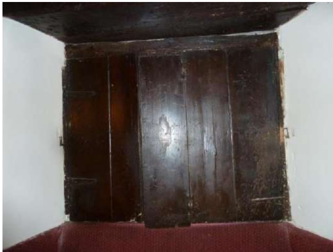
Original C17 Shutters to window nearest the fire
