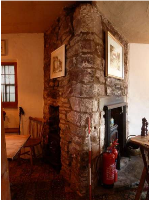
Corner Stone Chimney Stack[1 metre pole] Dividing wall removed
