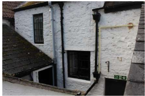
Rear of Southern GF gable
