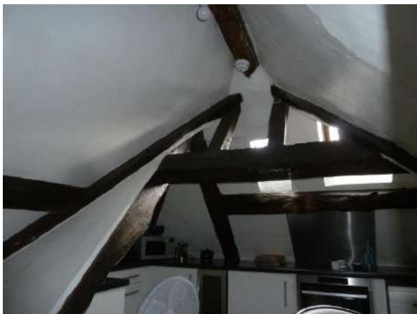
Exposed roof timbers of projecting hipped gable
