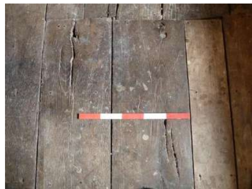
Original floor has wide boards [50cm scale pole]
