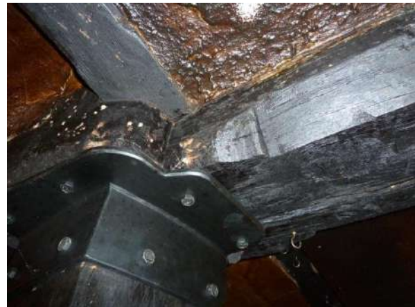
Post supporting chamfered beam with decorative stop
