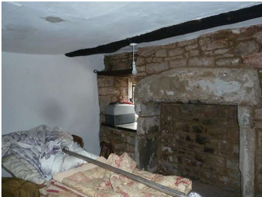
Stone Fireplace; square headed stone lintel with the suggestion of corbels with a moulding
