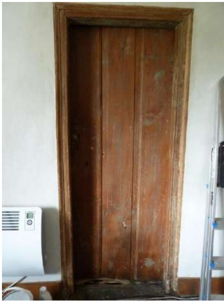
Original C17 Plank and batten door to Store
