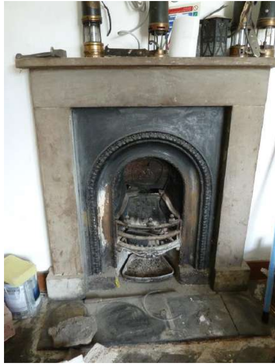
C19 cast iron fireplace
