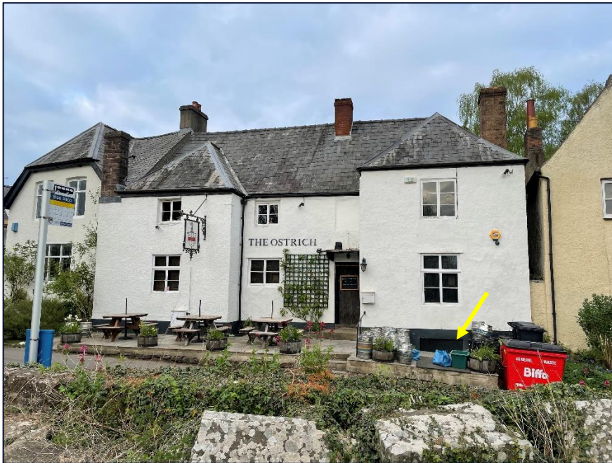
Figure 3A. Context: location of vertical plywood door to beer drop to the cellar (yellow arrow)
