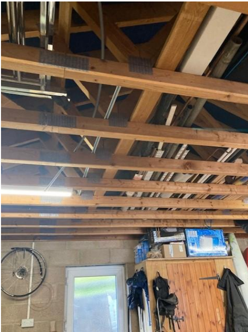
Fig. 11 – Garage roof structure
