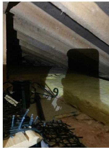
Figure 8 – Loft space in kitchen roof
