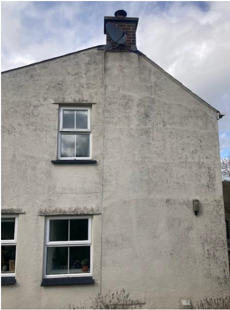
Figure 3 – South face of original cottage
