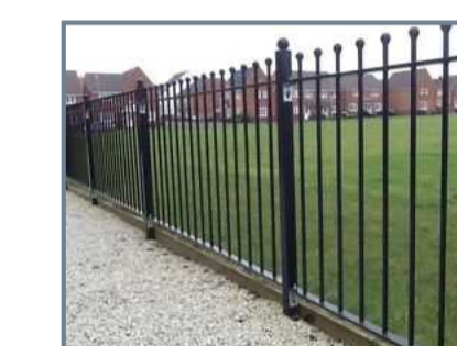
900mm high ball-topped railings with matching gate
