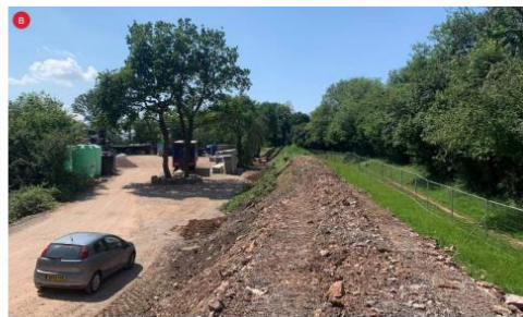
View B showing a similar view to view A but from the top of the bund and showing how it lines the edge of the site
