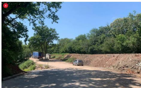
View from the access road showing the south of the 'Recycling Centre' site and the beginning of the bund
