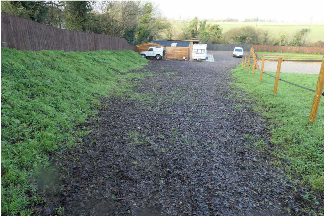
Photo 1, looking north across proposed works site area. Hardstanding and semi-improved grassland habitats present.
