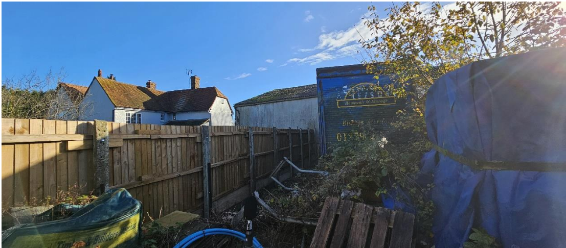
Fig.6: The northern end of the unit proposed for demolition (centre) seen looking east from the northern corner of the site, in context with the farmhouse (left).
