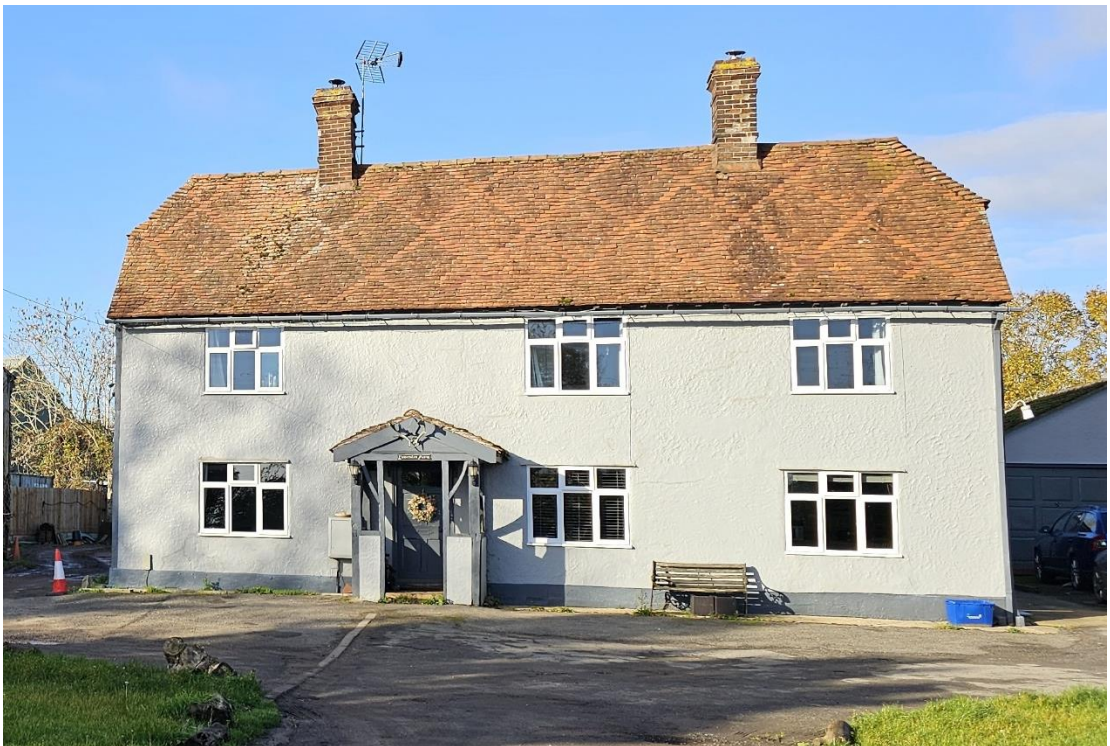
Fig.12: The principle southeast elevation of the farmhouse with render exterior and diamond pattern clay tiles to the half-hipped roof.
