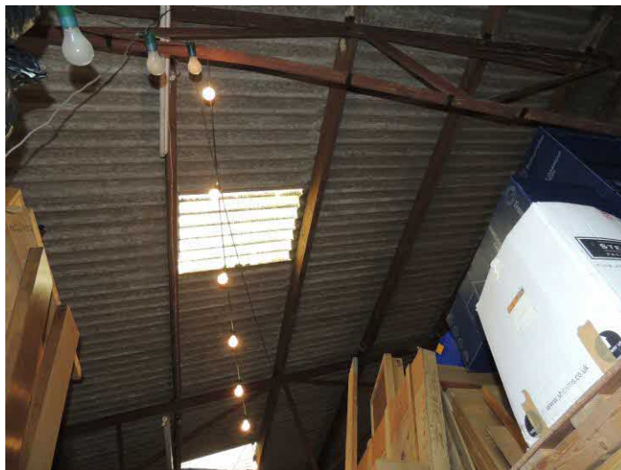
Photo 8: The roof had no features that might be occupied by bats
