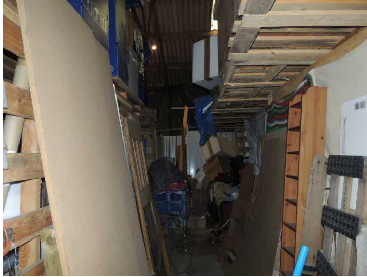
Photo 5: Interior of the barn
