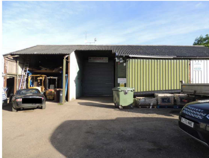
Photo 12: Light industrial unit to the north-west
