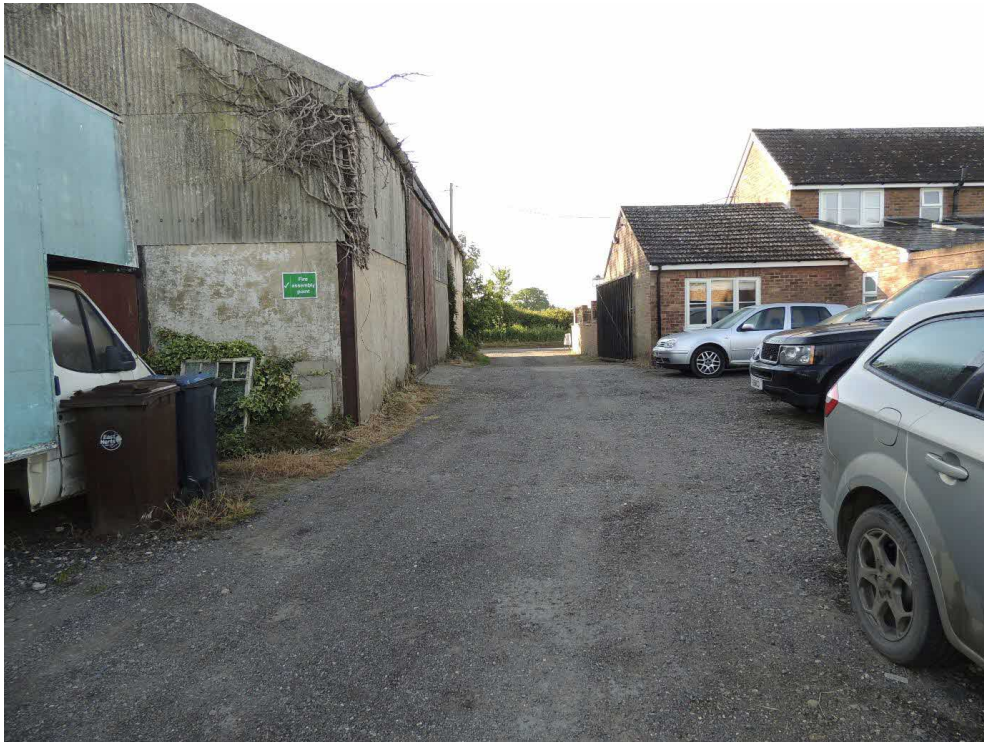
Photo 10: Looking south-eastwards from the survey building
