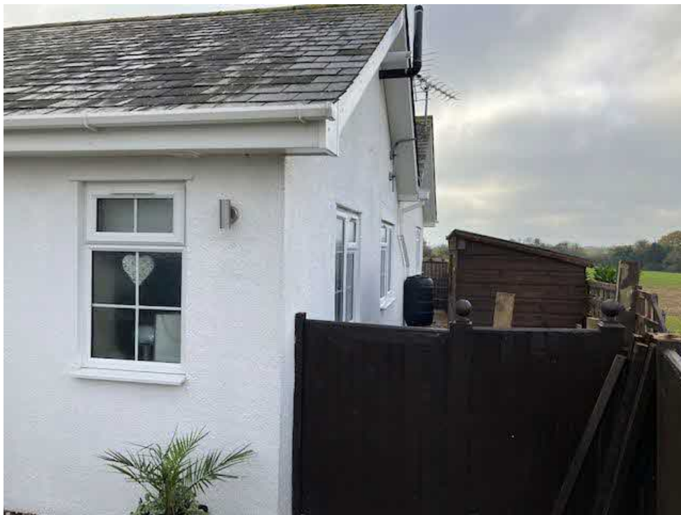
Roof Verges North West Elevation
