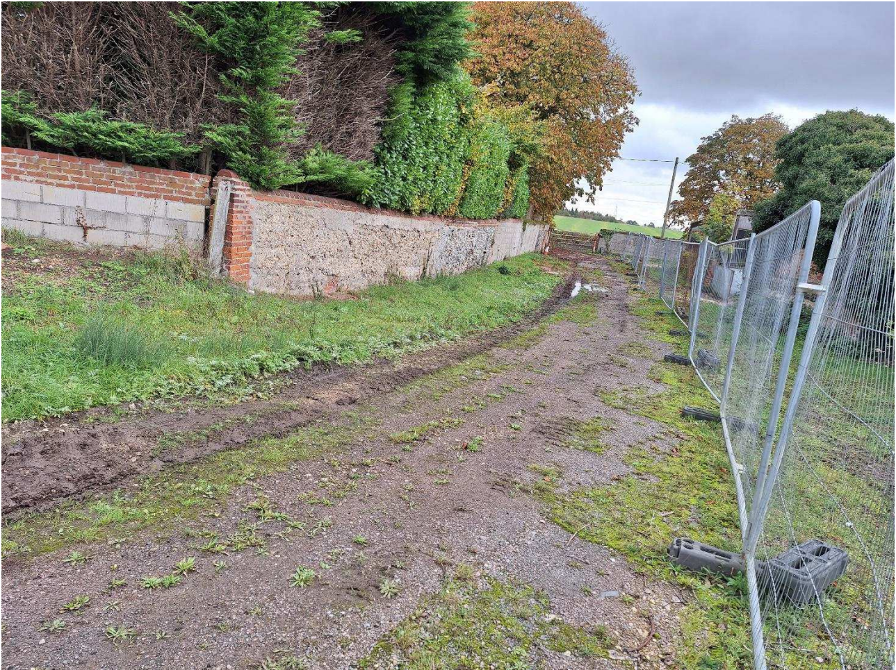
Access track, looking towards Wenden Road
