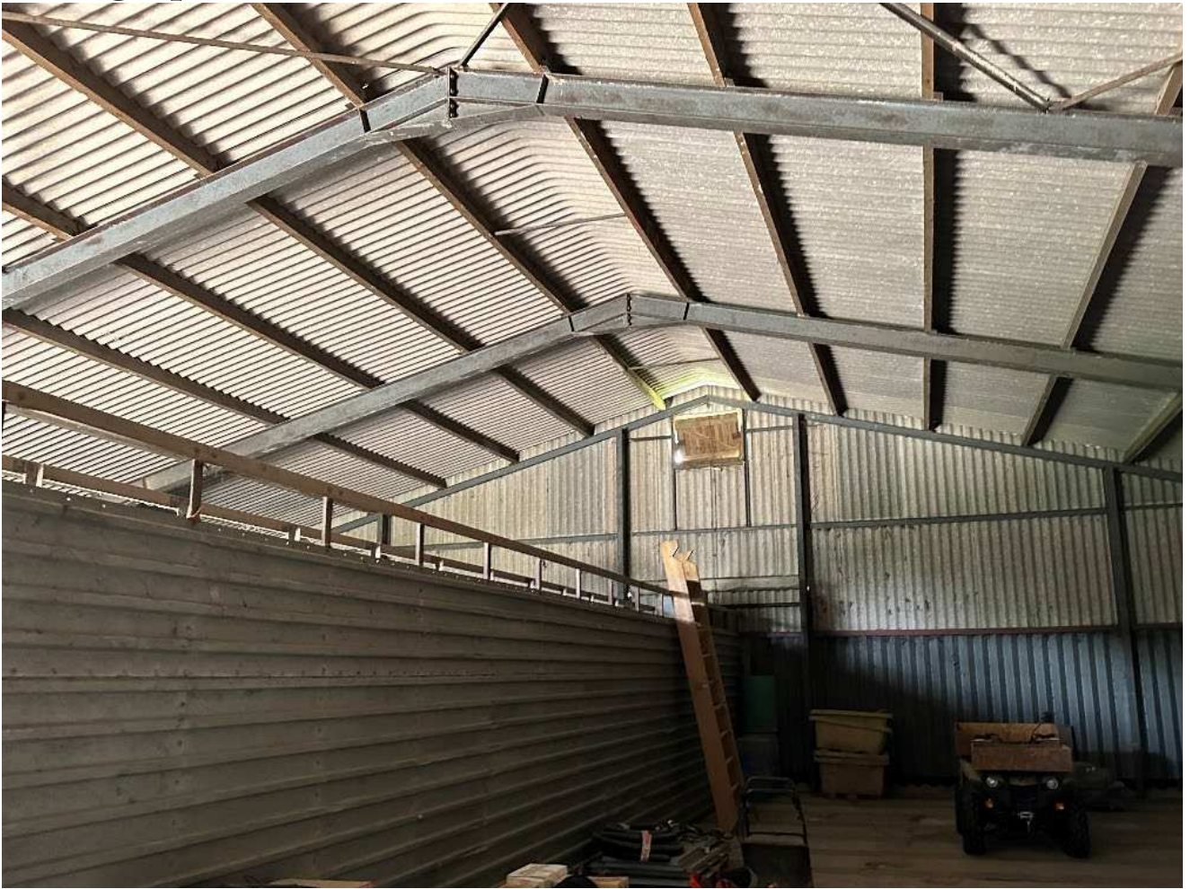
Internal view of Building 3.
