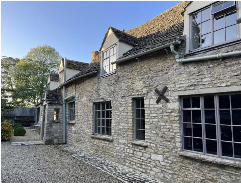
Figure 2: View of the southern elevation of the building.
