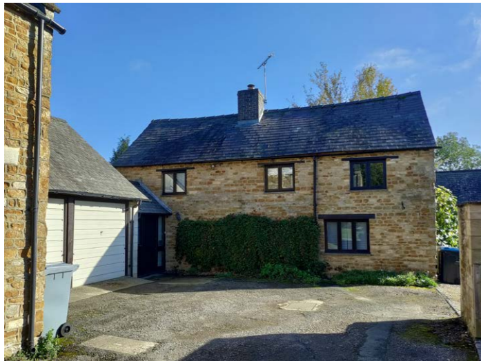
Existing Front (driveway facing) Elevation, viewed from the end of Chapel Lane
