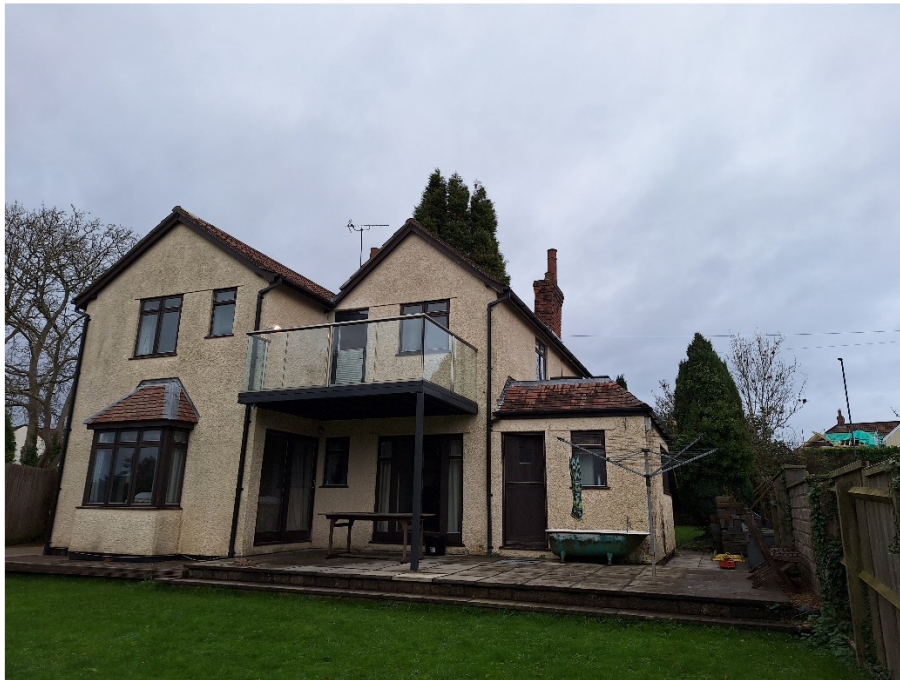
The balcony structure on rear of No 1 Old Aust Road
