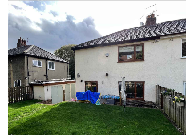
Photo 04 Showing North Facing Elevation
