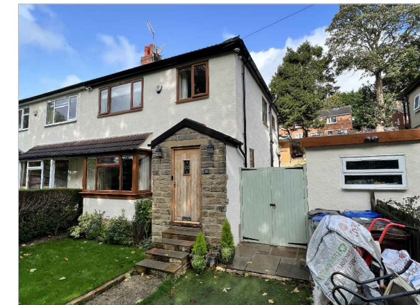
Photo 02 Showing South & East Facing Elevations
