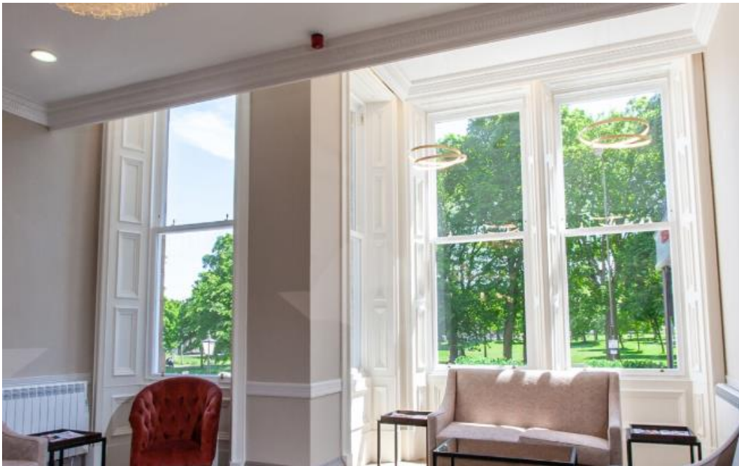
Fig 20: New timber sash and case windows (Blairs of Greenock)
