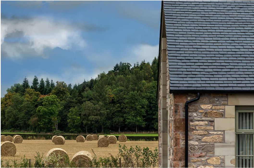
Fig 19: CUPA heavy 3 to match existing roof.
