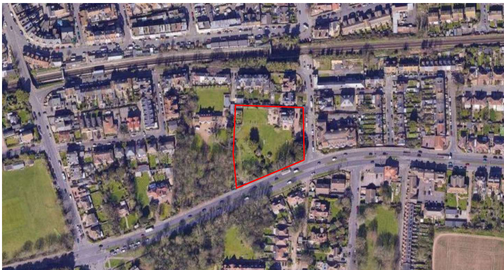
Aerial view of site
