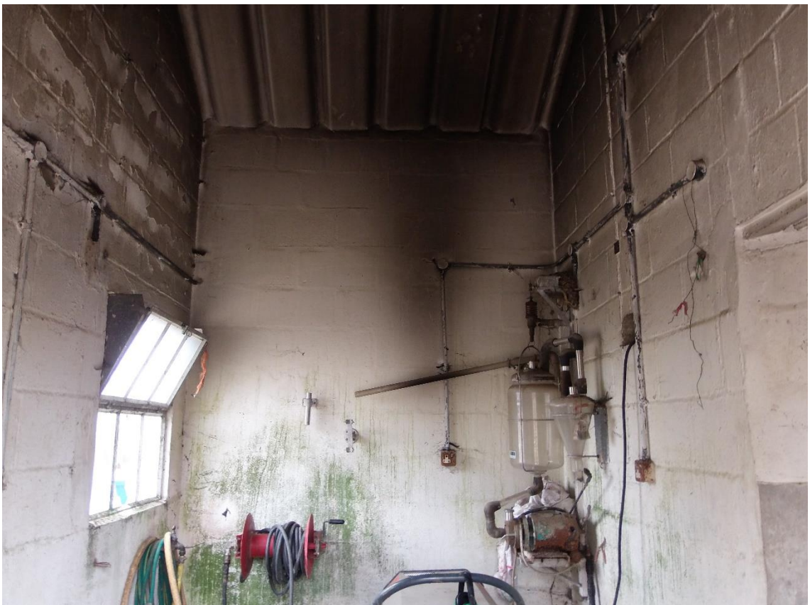
Photo 4 , internal view of section B.
