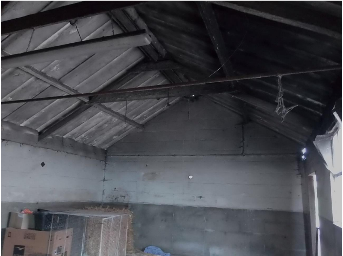
Photo 3 , internal view of section A.
