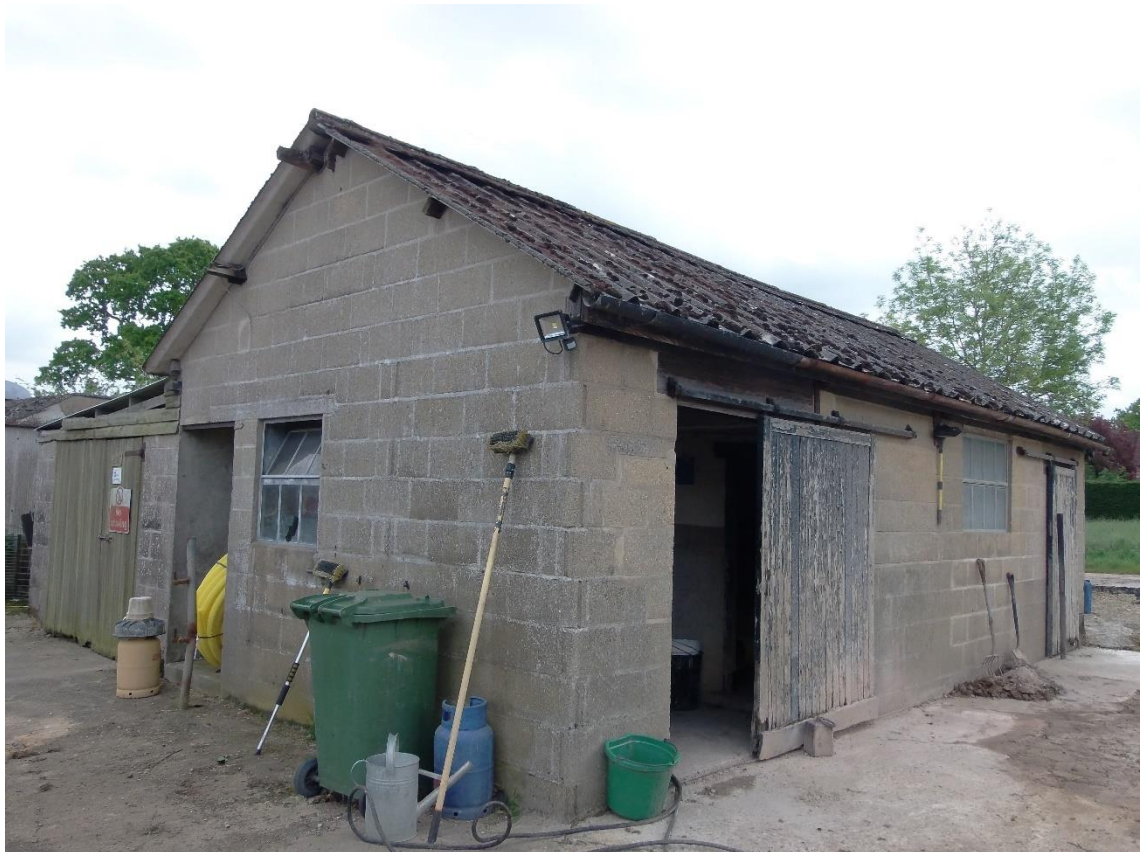
Photo 2 , north and west aspects of building one, looking southeast.
