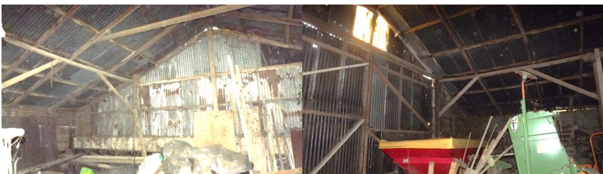
Fig 5 & 6. Internal view of west gable (left) and east gable and timber frame (right)
