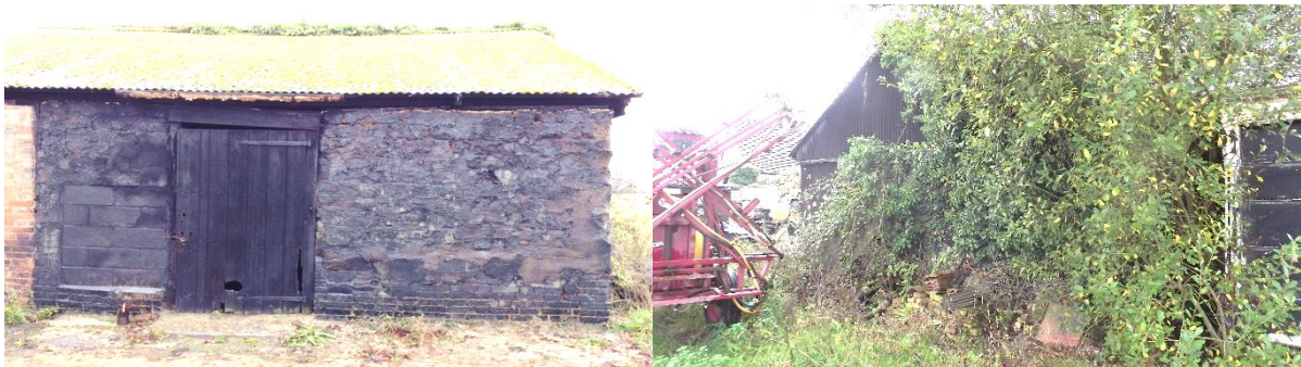
Fig 9 & 10. East elevation with tar coated clay lump (left) and overgrown north gable end (right)
