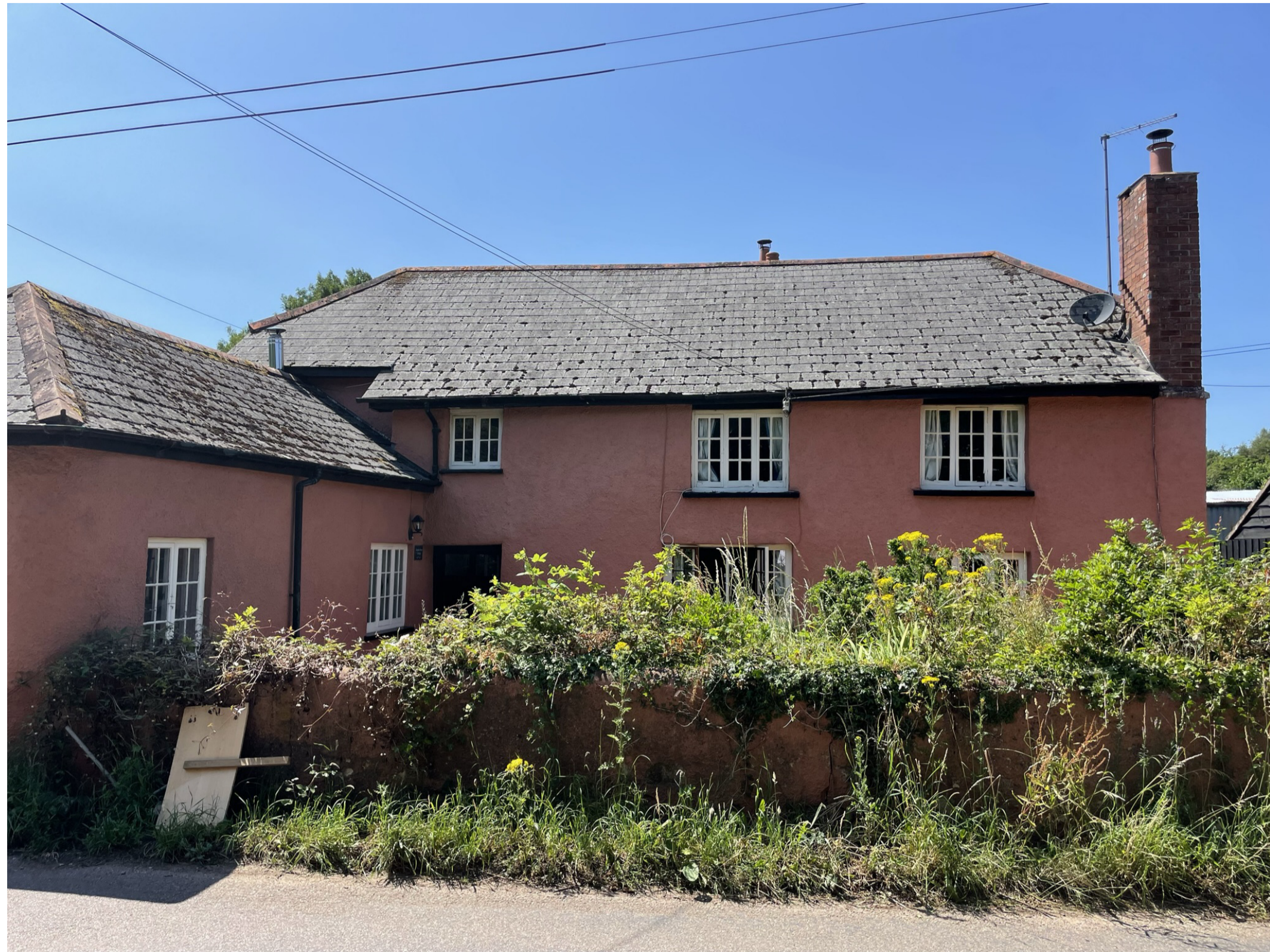
Photograph looking towards house (East elevation)
