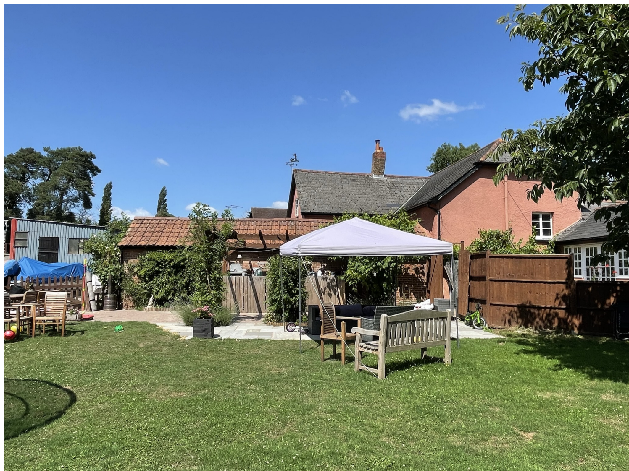
Photograph looking towards house (South elevation)
