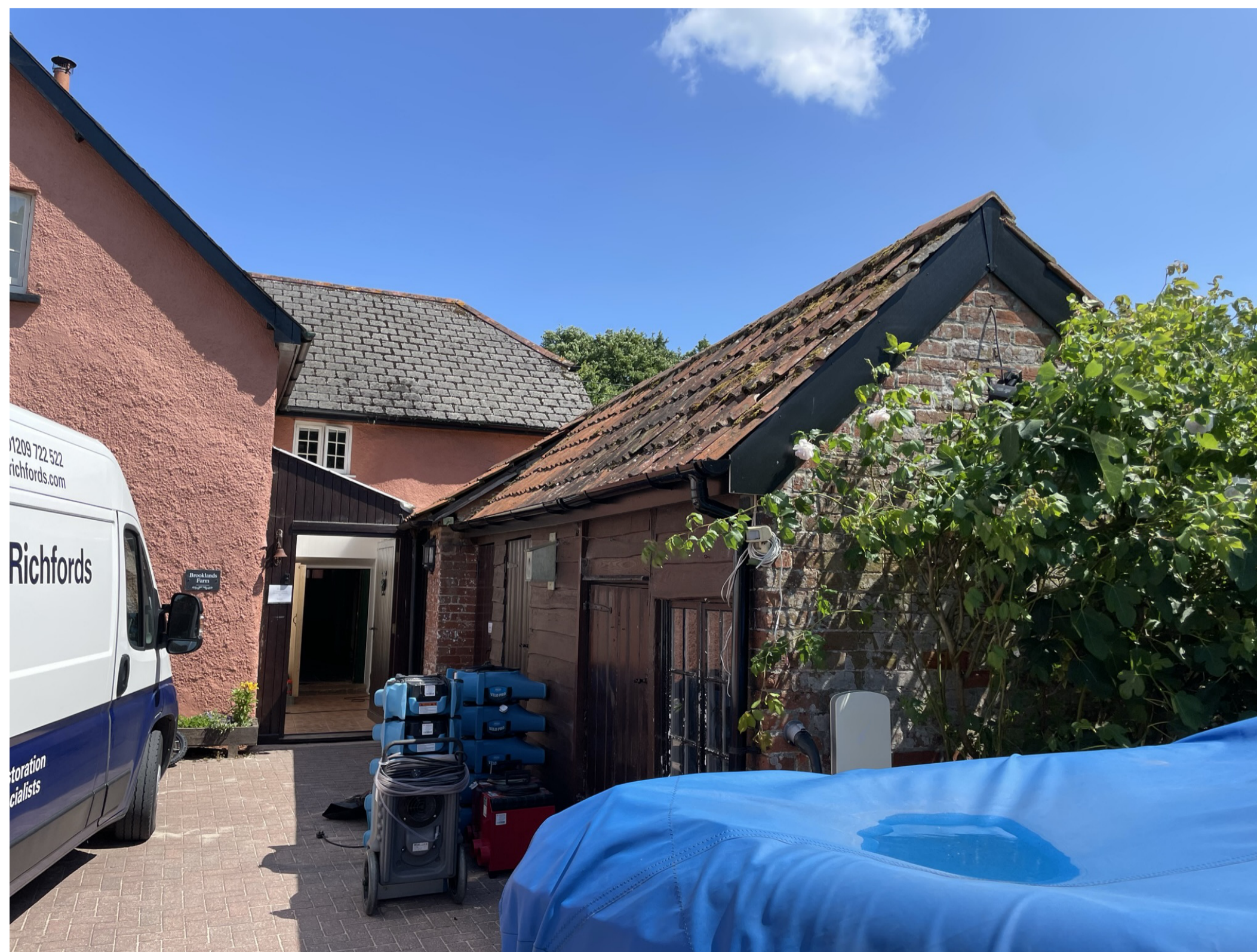
Photograph looking towards house (Part West elevation - showing rear entrance and structure to right hand side proposed to be demolished)
