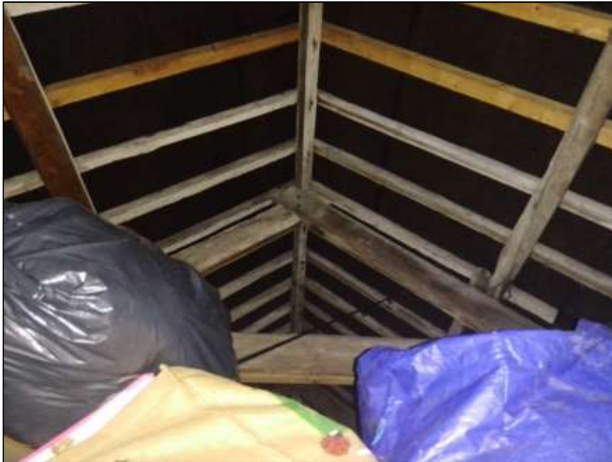
Photograph 2– View of the building interior.
