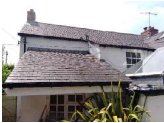
Photograph 2 – View of the north aspect.
