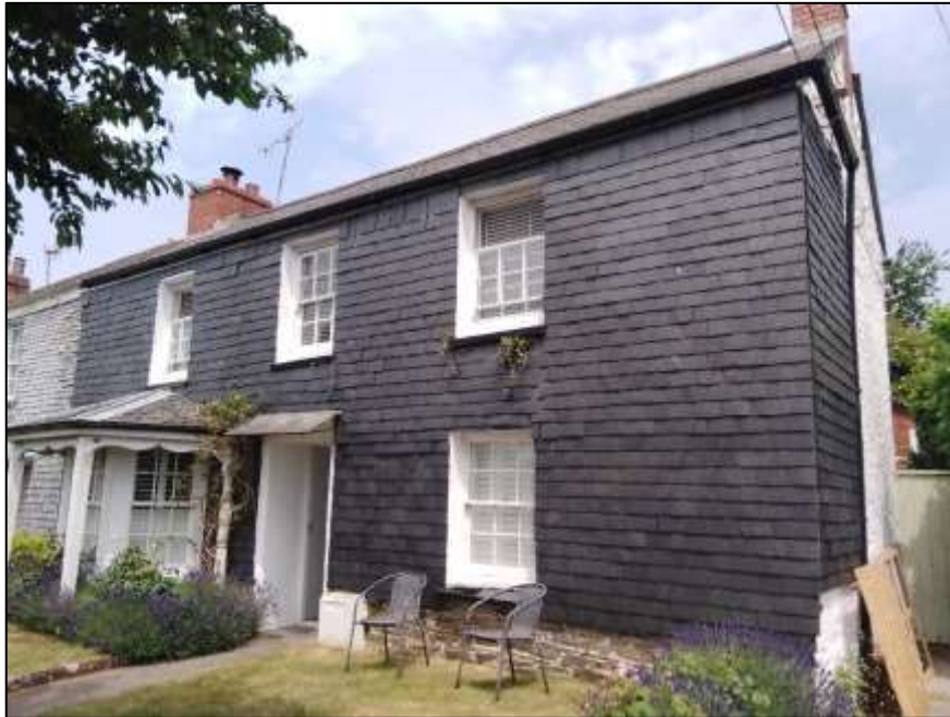
Photograph 1– View of the south aspect of the building.
