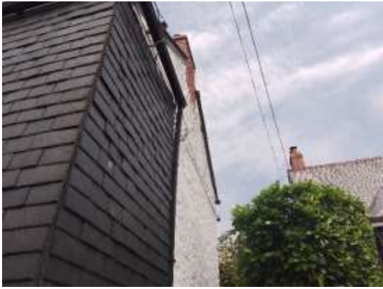
Photograph 1 – View of the east aspect of the building
