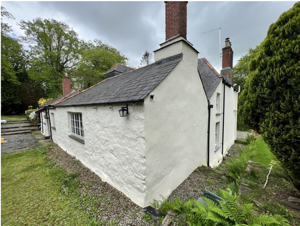
Figure 3 - Photograph showing North elevation.
