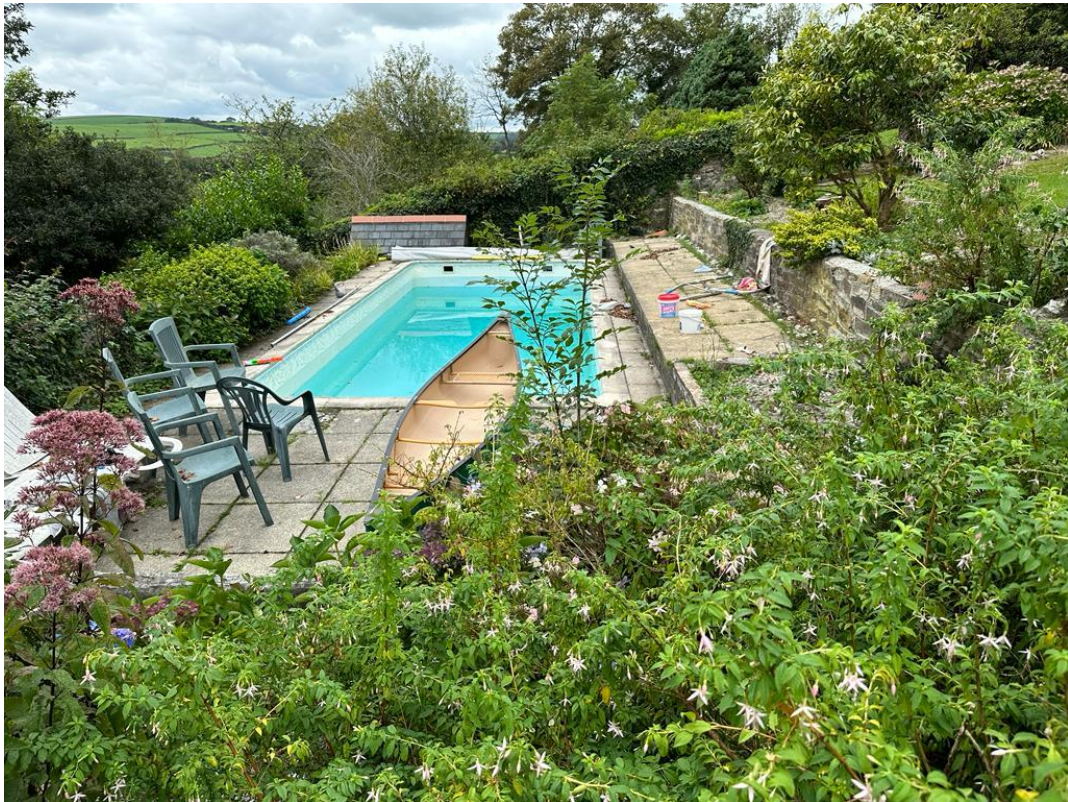
Figure 5 - Photograph showing existing pool.
