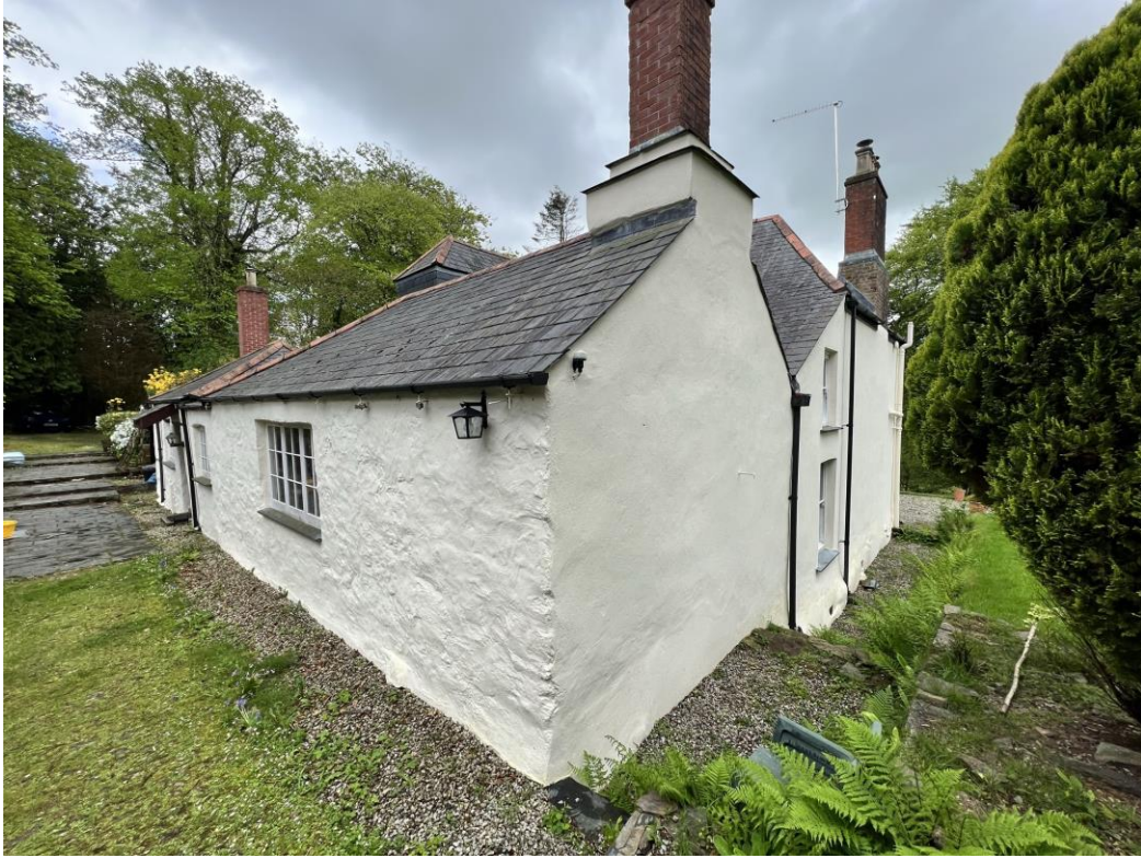
Figure 4 - Photograph showing North elevation.
