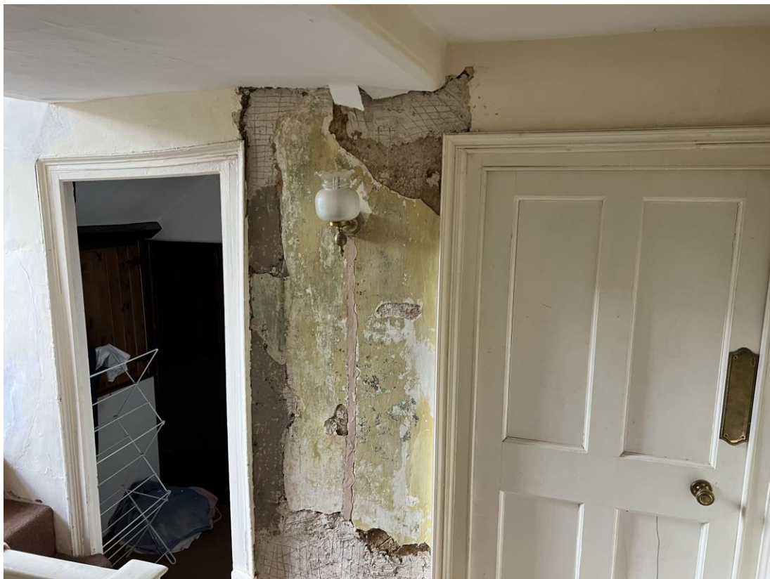
Figure 7 - Photograph showing area of wall to be replastered.
