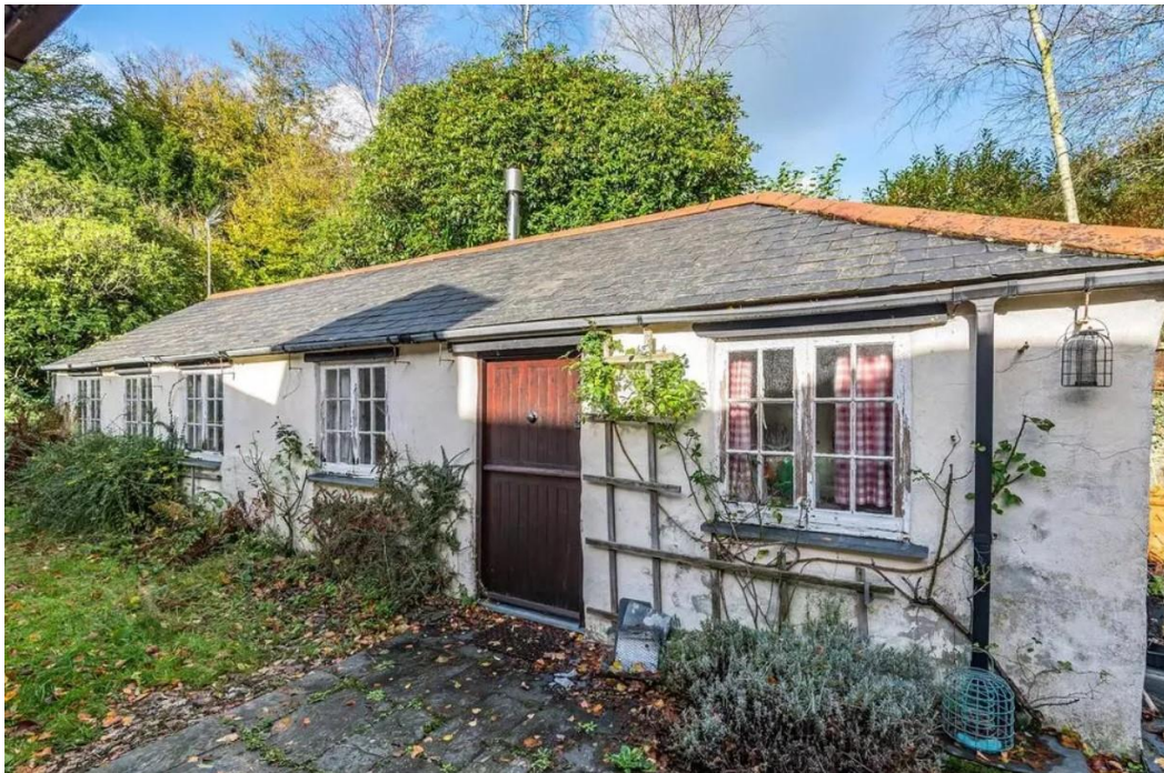
Figure 3 – Photograph showing Annexe South elevation.
