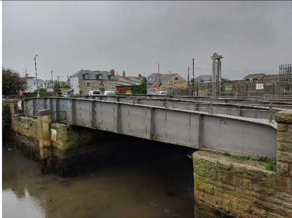
Pedestrian bridge – eastern face.
