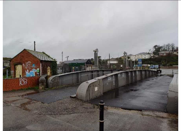
Pedestrian bridge viewed from south.
