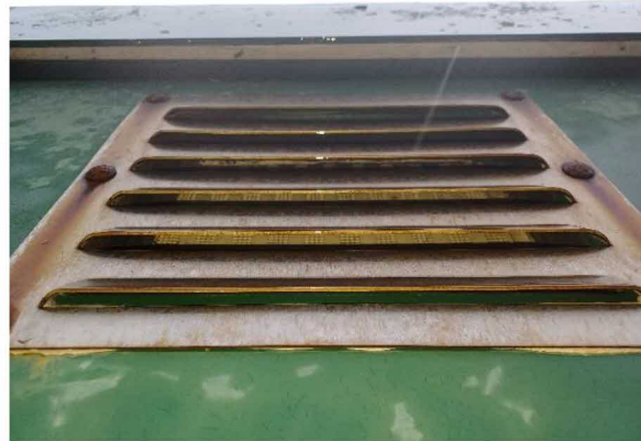
Vent and typical overhang on roof of kiosk.
