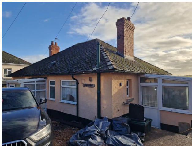
Photo 1: View northeast from front of 24 Mill Way; hipped roof, dual chimneys, PVC conservatory and porch
