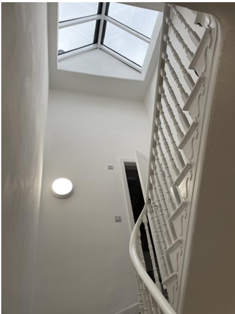
Plate 12: View of the stairwell rooflight as seen from first floor.
