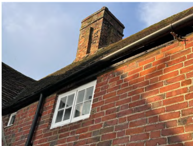
Figure 33: Externally visible wall plate
