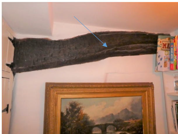
Figure 18: Possible door between Nos. 1 and 2
