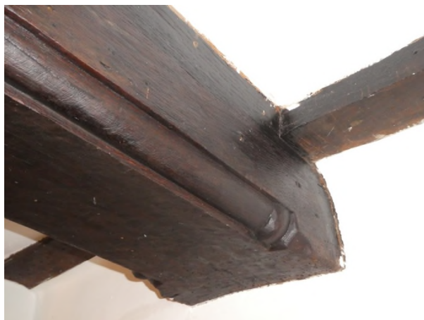
Figure 16: Axial beam with ovolo mouldings in the lounge
