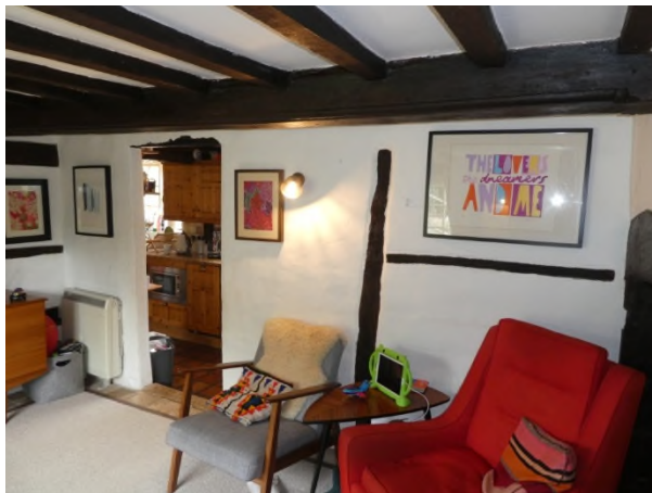
Figure 12: Timber framed partition subdividing the original ground floor room
