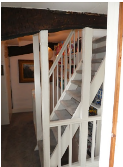
Figure 22: Ladder stair to the attic spaces
