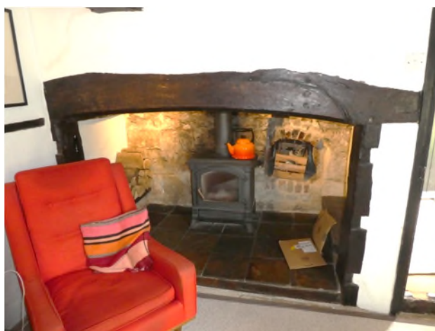
Figure 15: Fireplace with timber lintel in the lounge
