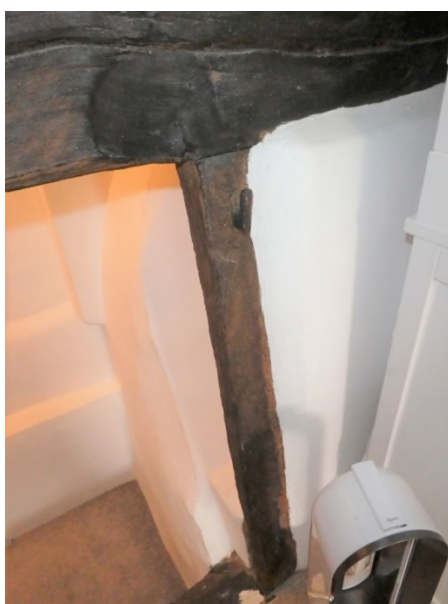
Figure 24: Iron pintles for a door into the attic space
