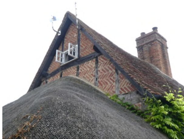
Figure 8: Queen strut truss with clasped purlins on the north-west elevation
