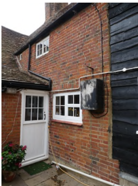
Figure 11: Rear elevation of the Phase 1 house
