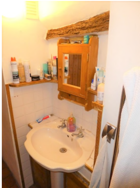
Figure 26: Recess in the bathroom that projects into the Phase 2 wing
