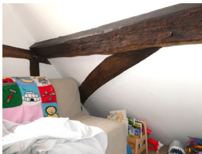
Figure 25: Curved windbrace in the attic bedroom
