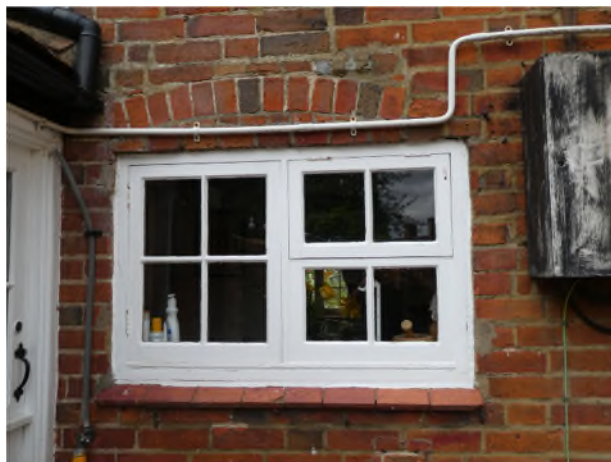
Figure 32: 20 th century window in an enlarged opening on the rear elevation of Phase 1
