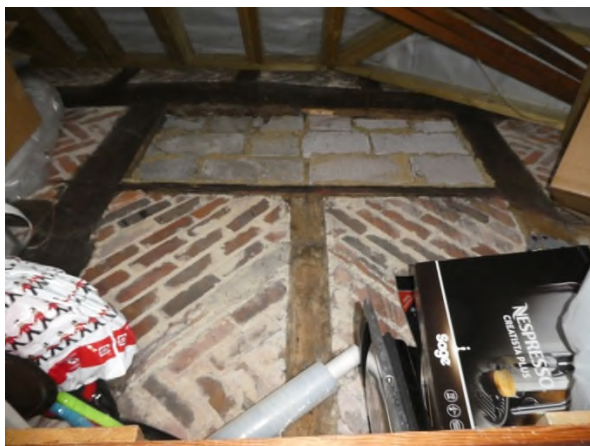
Figure 9: First floor window opening on the original north-west elevation viewed from the roof void over the dining room
