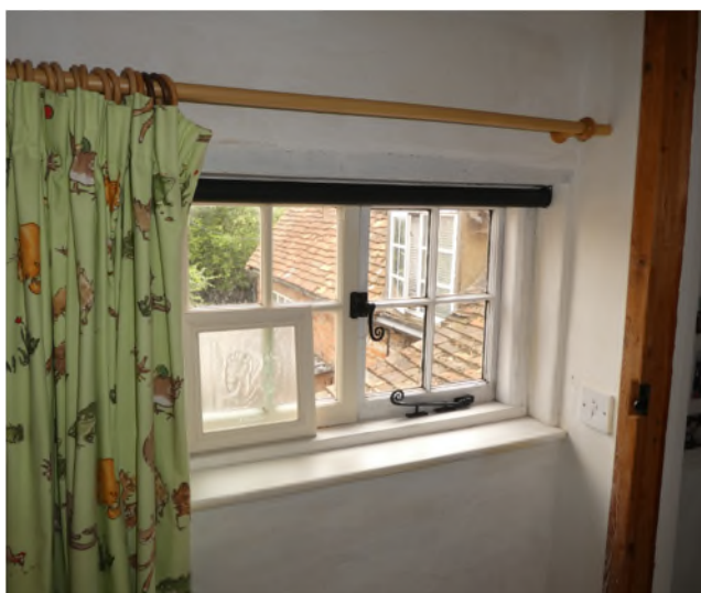
Figure 34: Casement window on the rear elevation of the first floor
