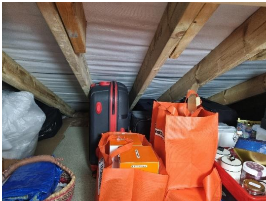
Photo 5 – main void in the eaves
