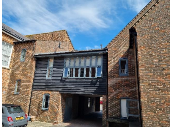
Photo 2 – west facing elevation
