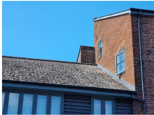
Photo 4 – composite roof tiles, east facing elevation
