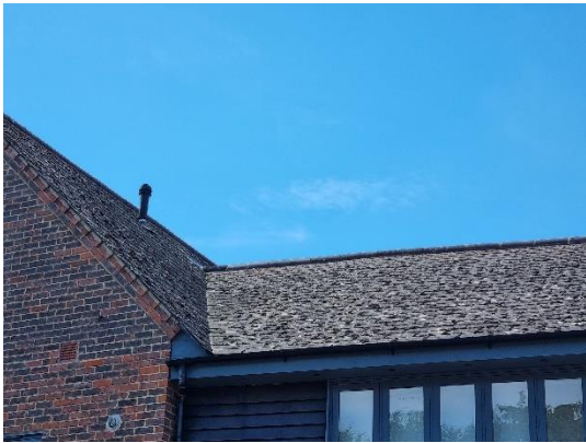
Photo 3 – composite roof tiles, east facing elevation
