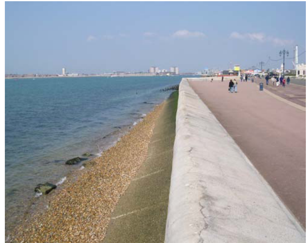
Sea wall at Southsea, Portsmouth.
